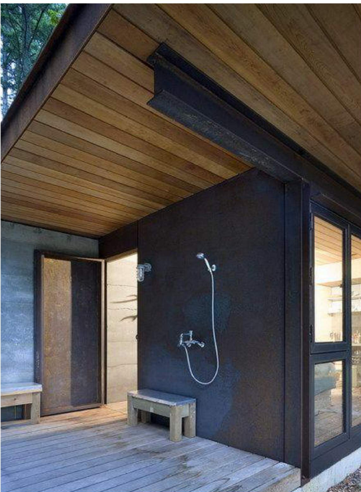
STEEL DETAILING / WOOD CEDAR SOFFITS
