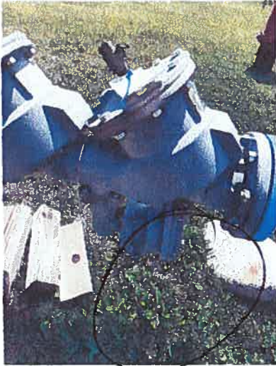
Water backflow controls in front of baseball field, has a small, but persistent dripping under the number 4
