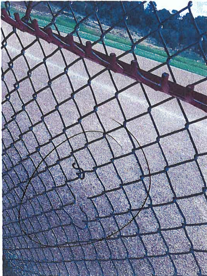
Inside the dugout, chain link has been cut and sharp pointy edges protrude on both sides under the bat-holder hooks
