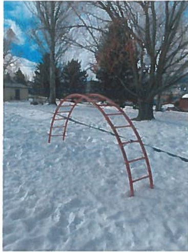
Bent Climber- To be replaced by a spin element
