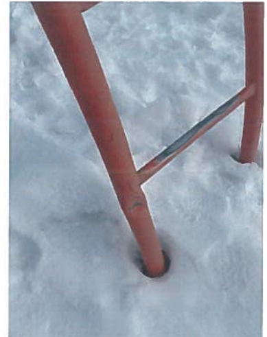
Bent Climber- To be replaced by a spin element
