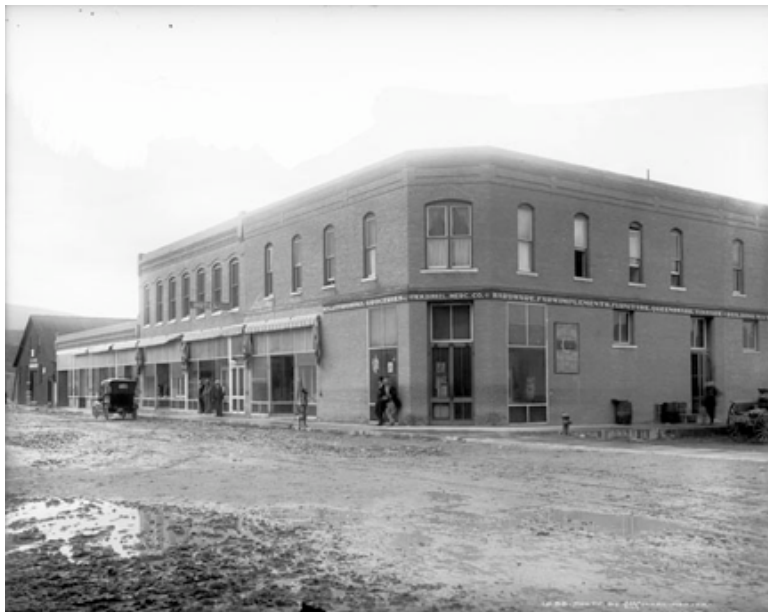
Figure 8 • The Dinkel Building
