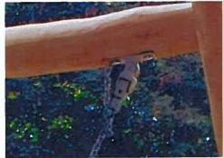
Swing hangers for Robinia wood crossbeams are made of stainless-steel brackets and can move over two axis. The plastic flange bearings are silicone enriched to make the suspension maintenance free.
