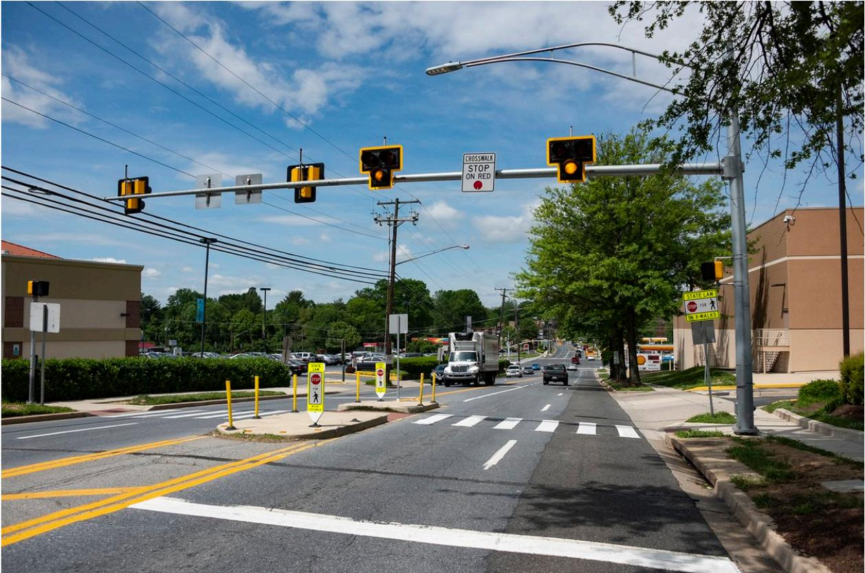
Figure 17: Pedestrian Hybrid Beacon (PHB)
