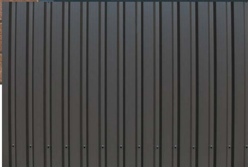
3 BRONZE CORRUGATED METAL SIDING WITH EXPOSED FASTENERS
