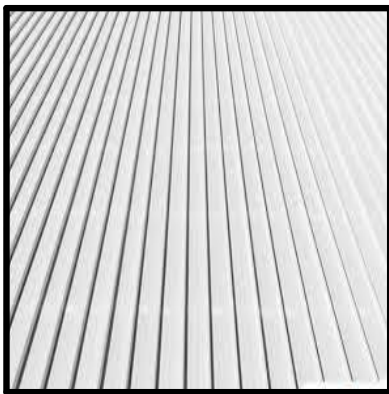
mtl-1 standing seam metal roof
