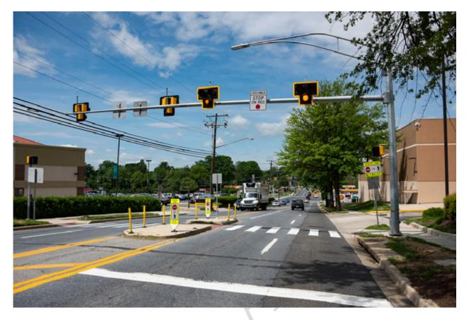
Figure 17: Pedestrian Hybrid Beacon (PHB)
