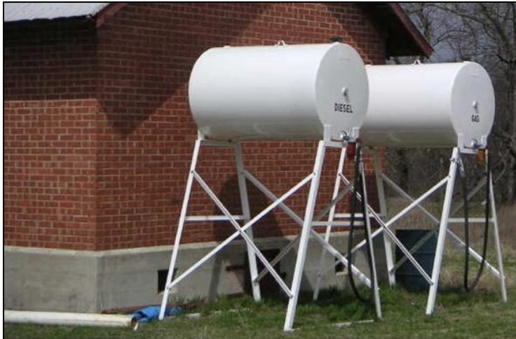
Figure 29: Example fuel storage tanks with no secondary containment Source: duboisswcd.org
