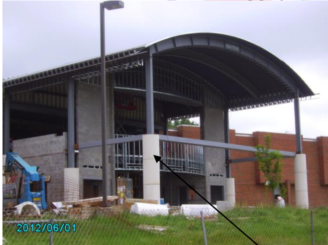
column covers being installed
