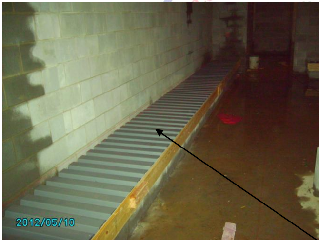
Steel decking used as form for concrete benches
