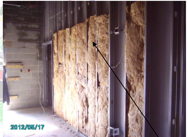
batt insulation between sheet rock walls
