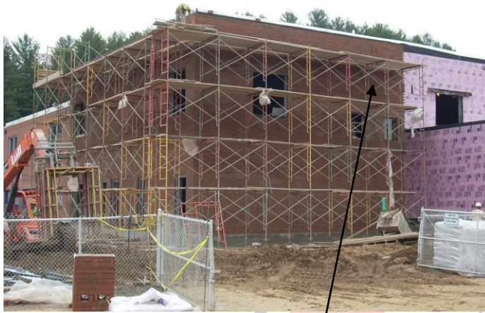
Exterior brick being installed
