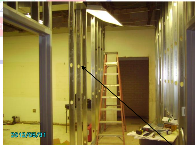
new stud framing and door frame at existing
