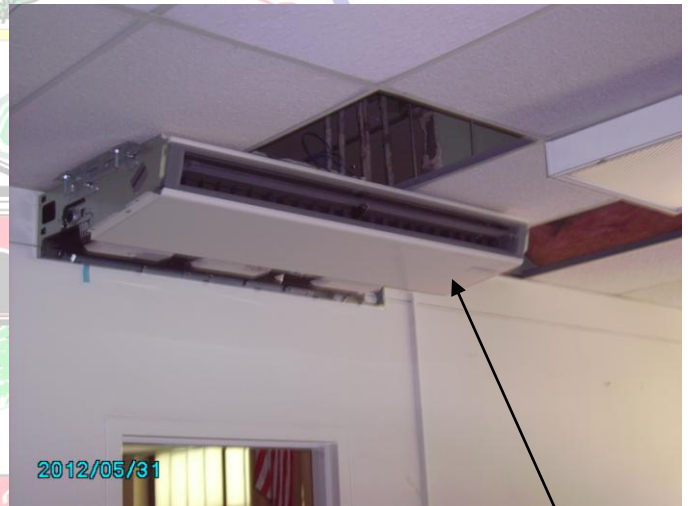
New in-room HVAC unit at ceiling
