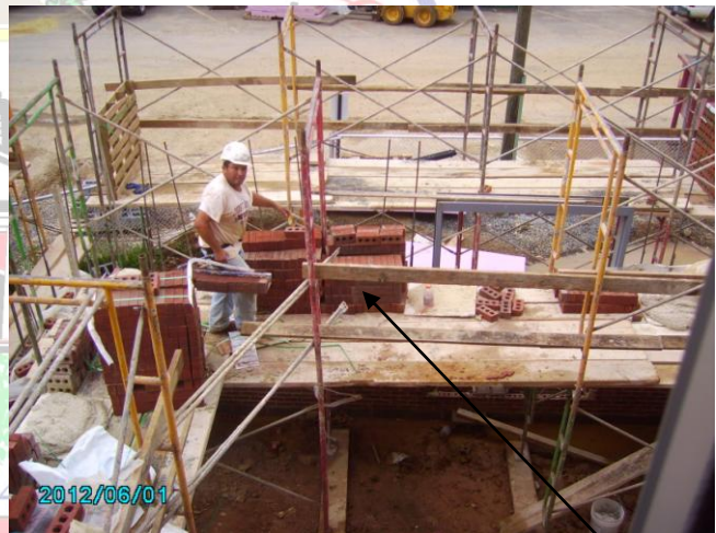
Mason working on Patio at weight room
