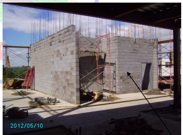
toilet area, elevator shaft and bearing walls for steel
