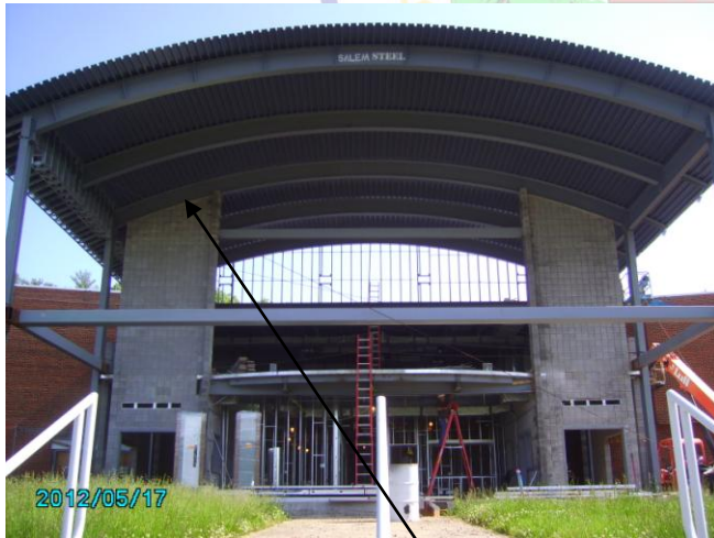
CMU to underside of deck
