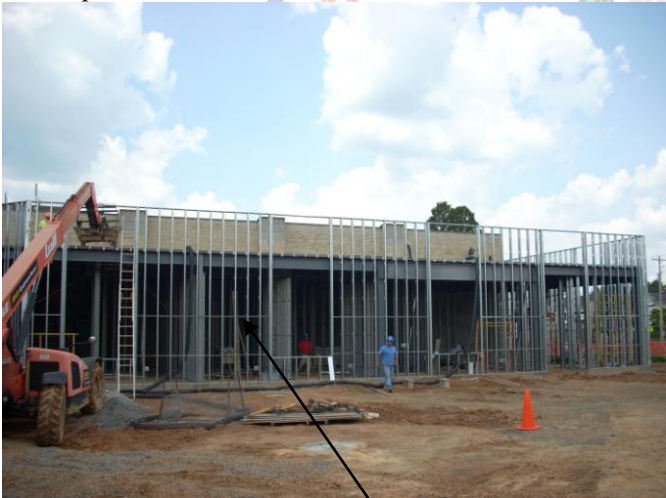
Exterior steel framing
