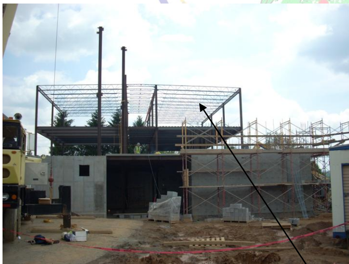
Steel columns, decking and beams
