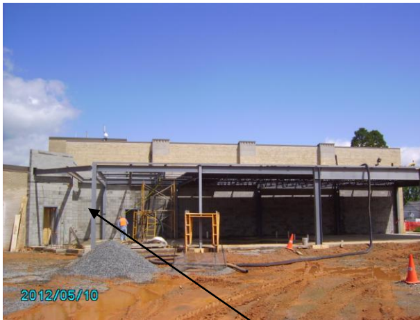
Masonry block walls
