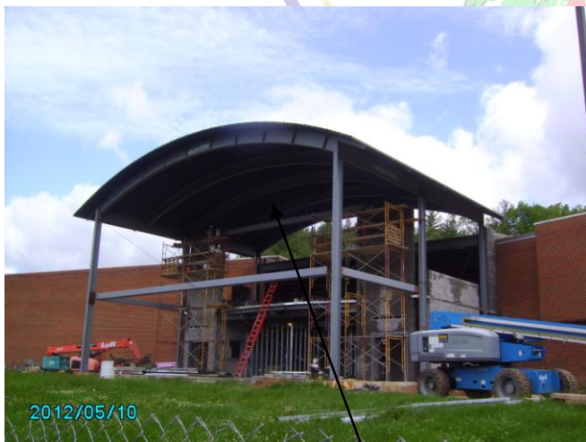
Steel decking at barrel roof
