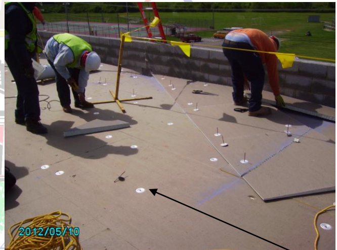
Polyiso roof insulation mechanically fastened
