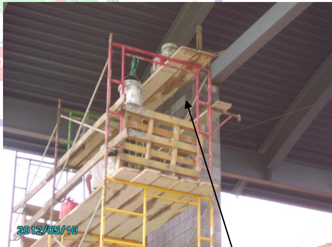
mason finishing block at steel deck
