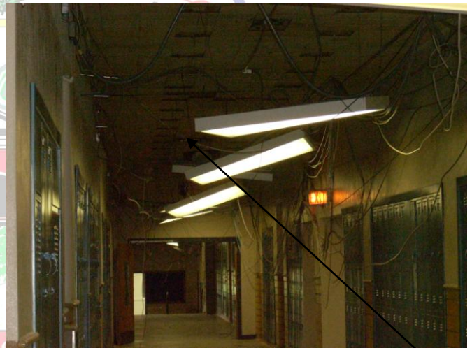
demolition of existing corridor ceilings
