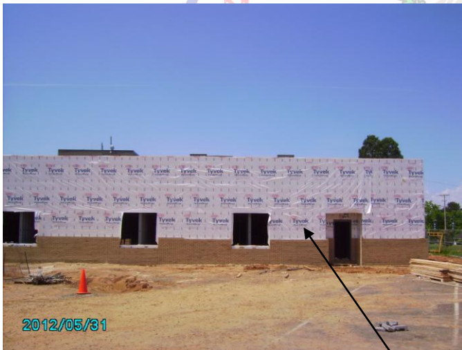
Exterior building wrap and new brick
