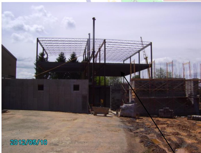
Roof bar joist and metal decking
