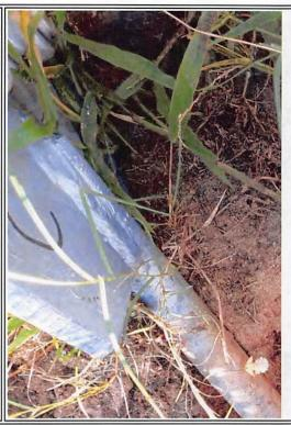
F. Anchors Do Not Have Cathodic Protection. We Recommend Furnishing And Installing Cathodic Protection.
