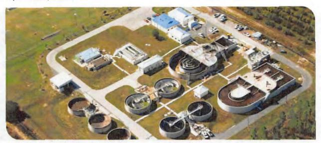
Halff provided design, permitting, and construction administration services for the Woodlea Road Water Reclamation Facility expansion. This project expanded an existing facility from 1.0 mgd to 3.0 mgd, upgrading to tertiary treatment to supply reclaimed water. The treatment process provides biological nutrient removal of nitrogen through a modified Ludzack-Ettinger process utilizing anoxic basins and oxidation ditches. The new facility design incorporates the following features:
