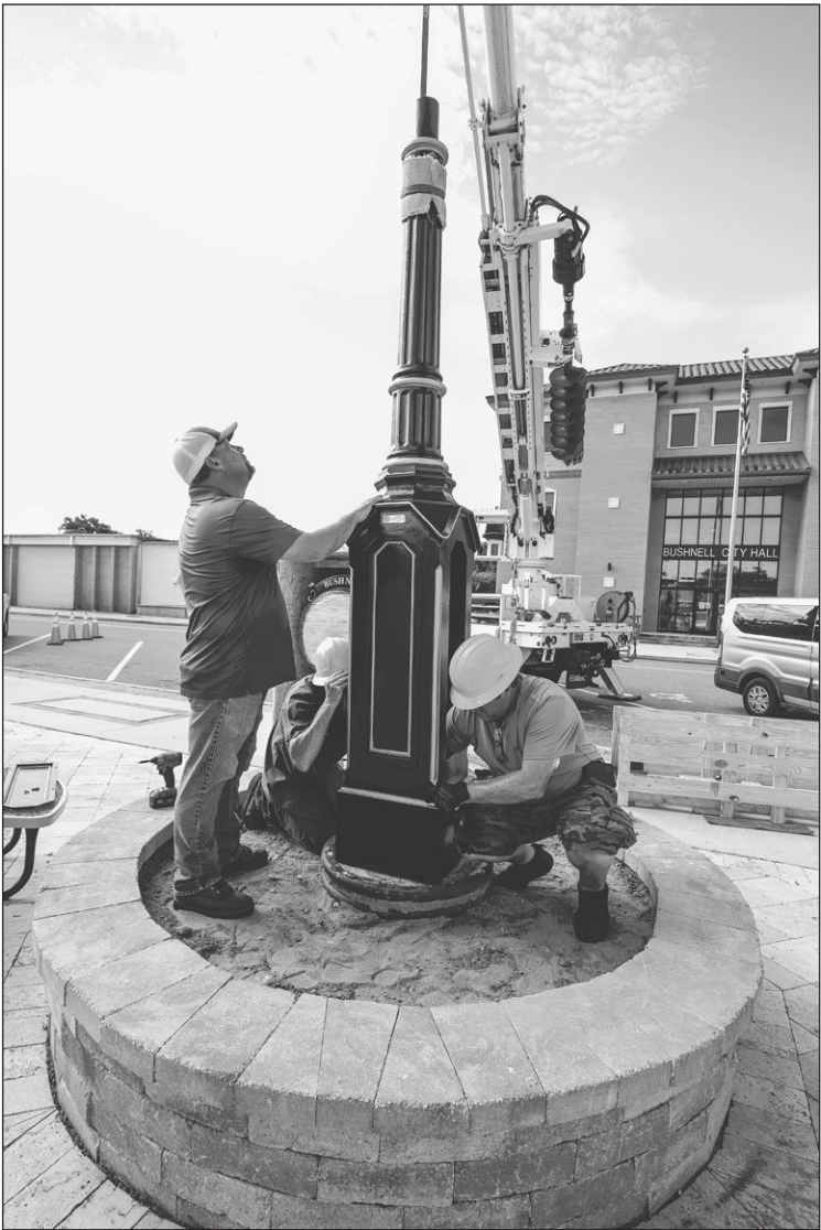
Bushnell Public Works staff and contractor for the Verdin Company guide the 700-pound cast iron base and post assembly into place as the clock installation gets underway.
