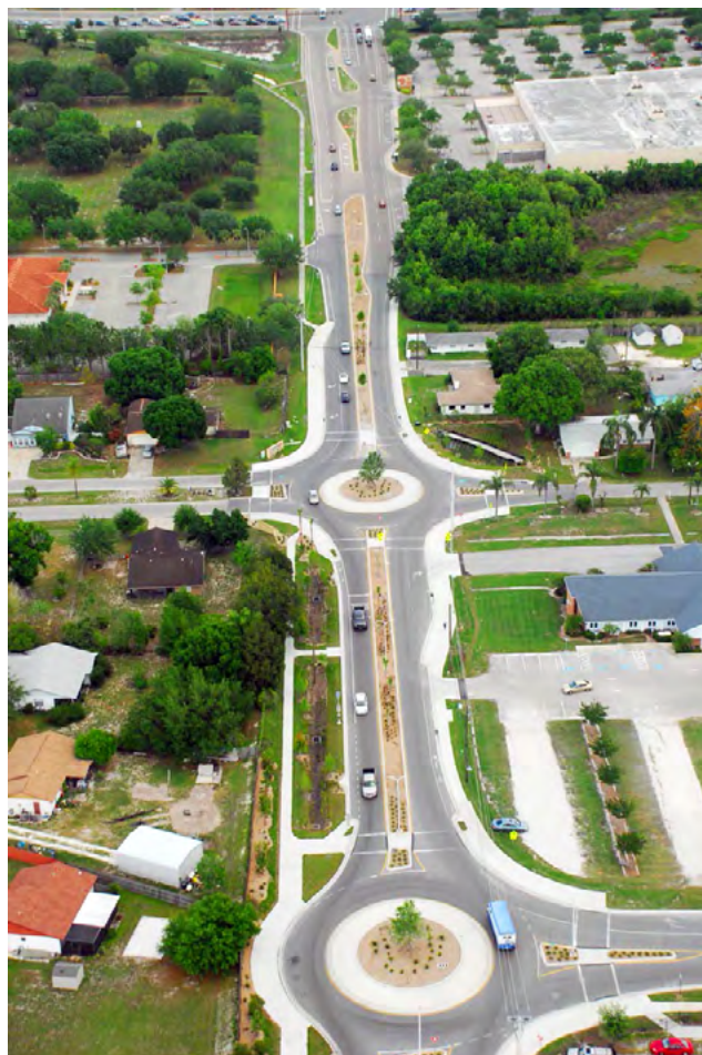
Figure 7-14: This is an example of a series of roundabouts serving a median divided roadway (Source: Stantec)
