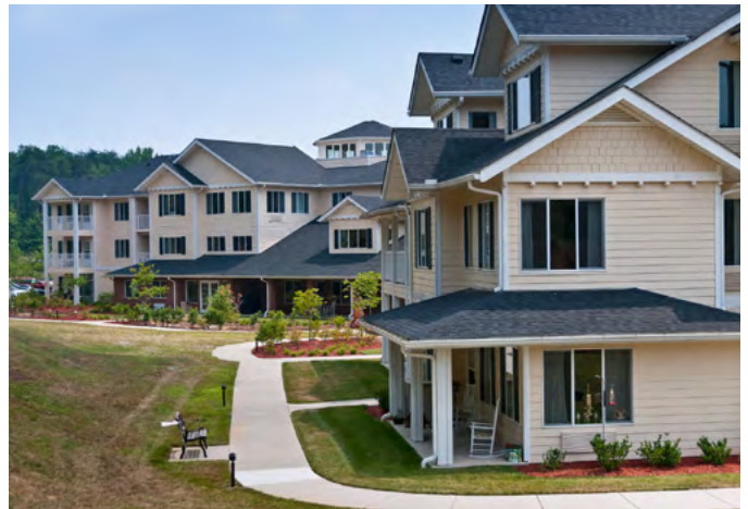
Figure 6-4: Evaluating development proposals on a variety of criteria including pedestrian connections and proposed landscaping will help the City to maintain its residential form. (Source: Stantec)
