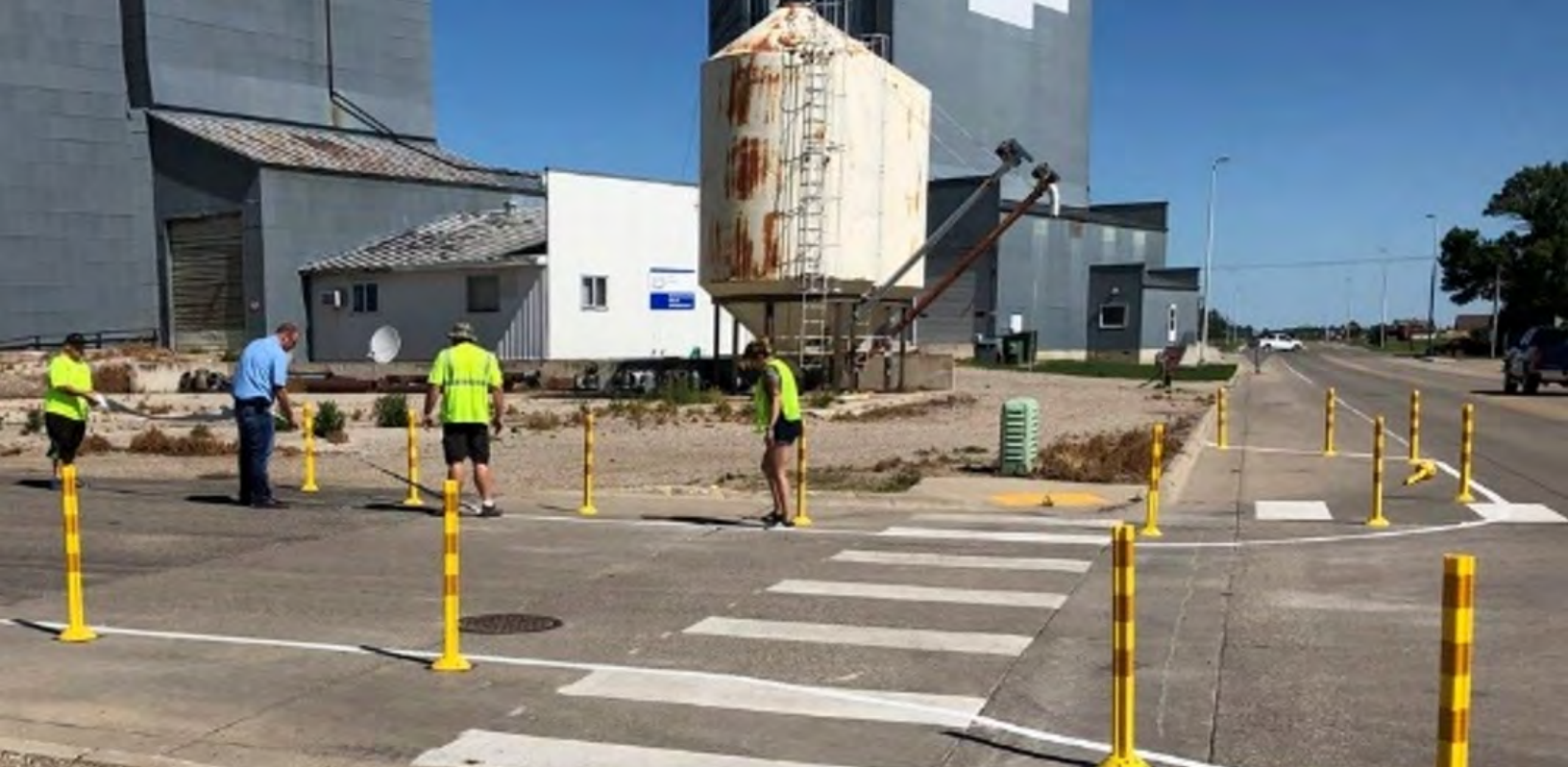
A roadway demonstration used bollards to create temporary bump-outs at the intersection of Main Street and Center Avenue, with the intention to increase driver awareness and improve pedestrian safety.
