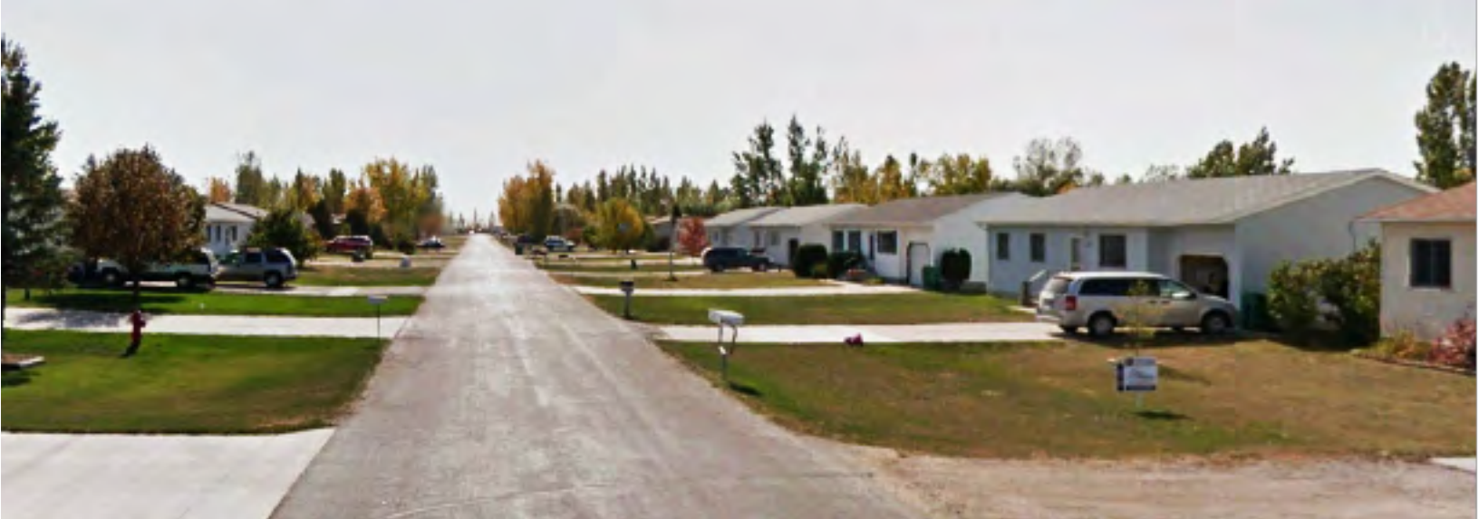
There was significant development in Horace in the 1960s. The supporting infrastructure is sometimes limited, with some streets lacking sidewalks and storm sewers. (Source: Google)
