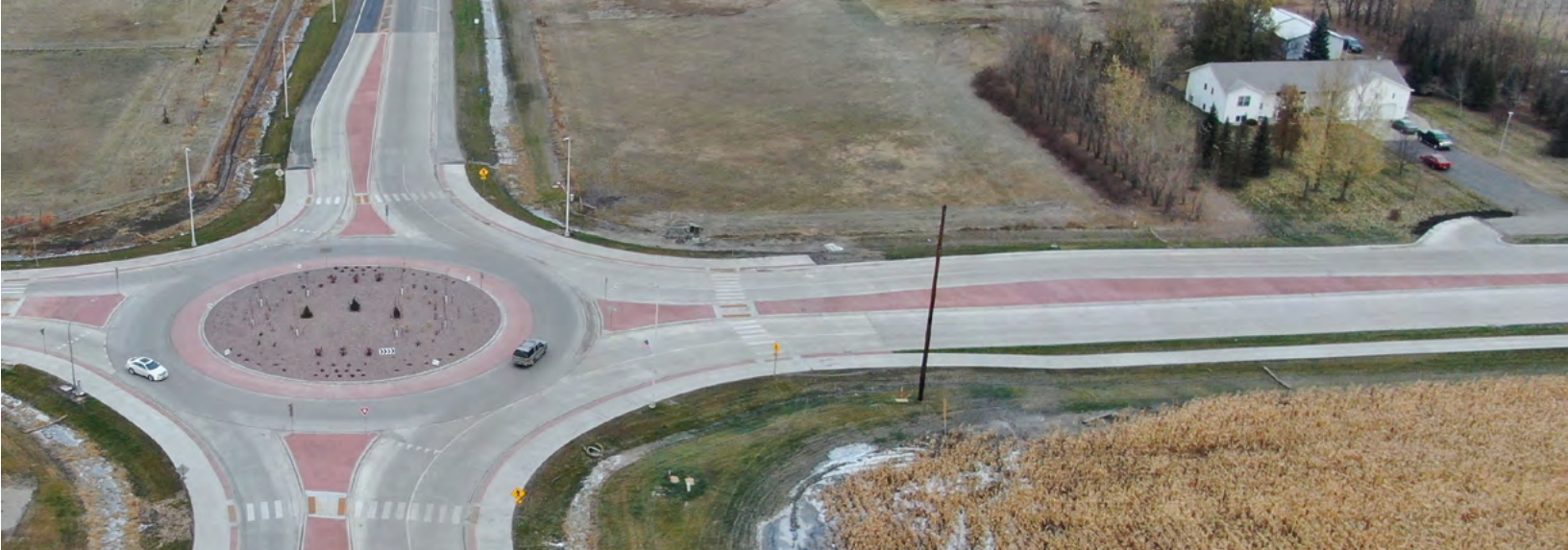
A recently completed roundabout in Horace improves mobility and safety
