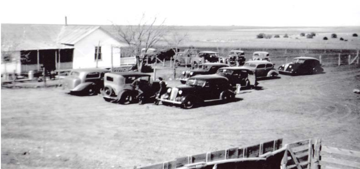
Photo courtesy of Brad Hill.
