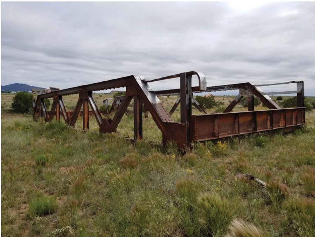
Trestle bridge, awaiting installation across Bachelor Draw. Photo Courtesy of the Town of Edgewood Parks and Recreation Department.
