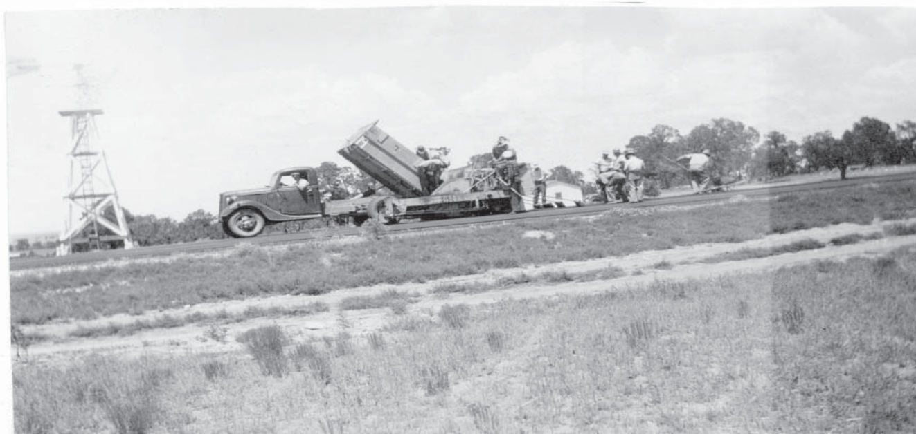
C. Brad Jones/Ann Jones/Dick Jones pavement crew. Photo source unknown.
