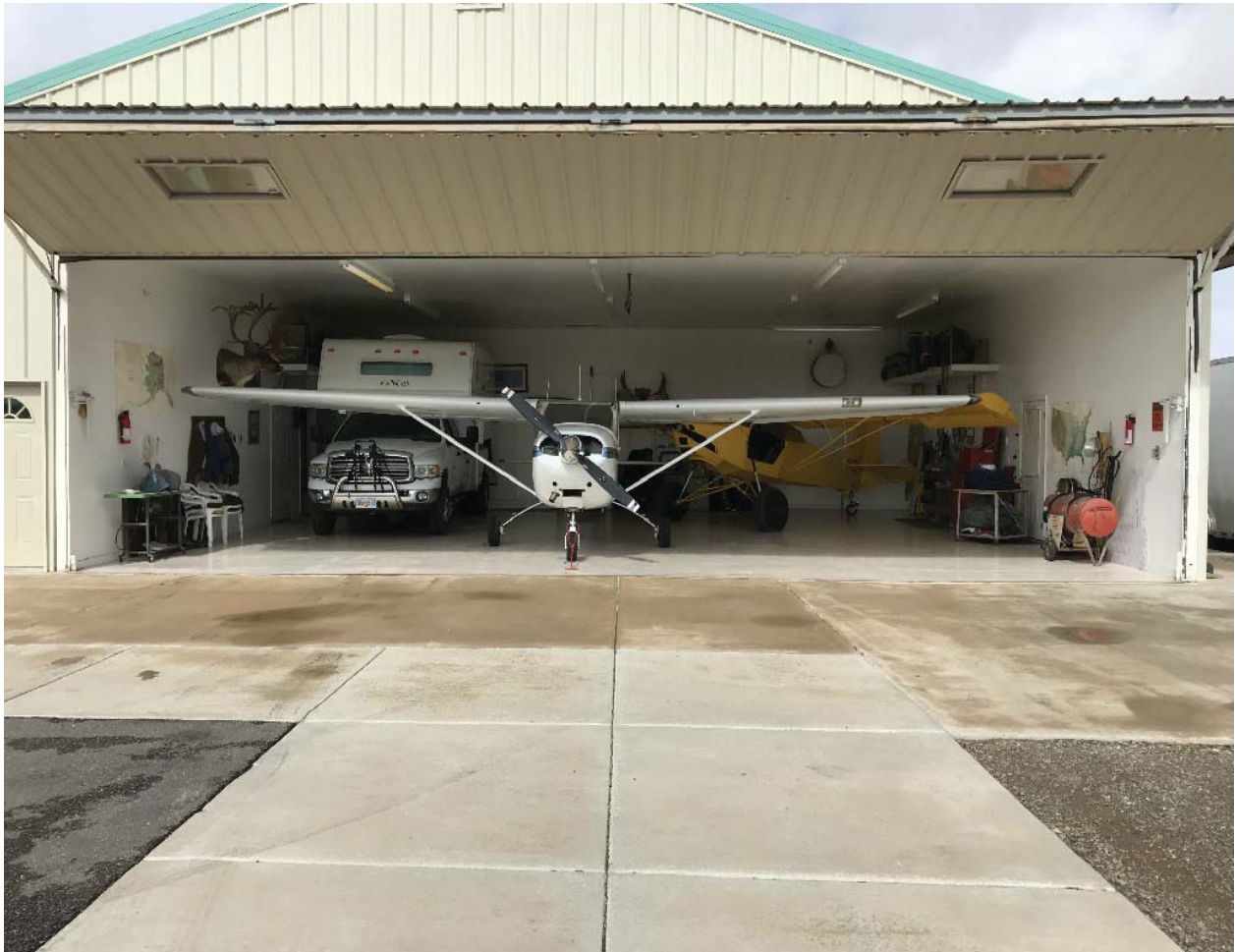
Sandia Airpark Hangar. Photo courtesy of John Bradley.
