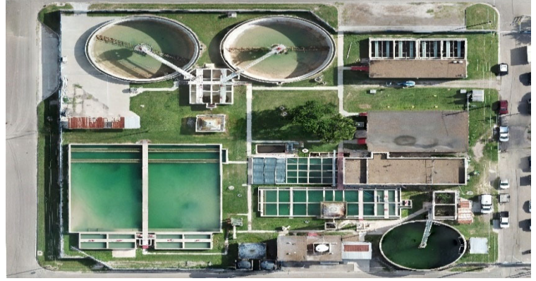
DOWNTOWN WATER PLANT - 500 E. MAHL.
