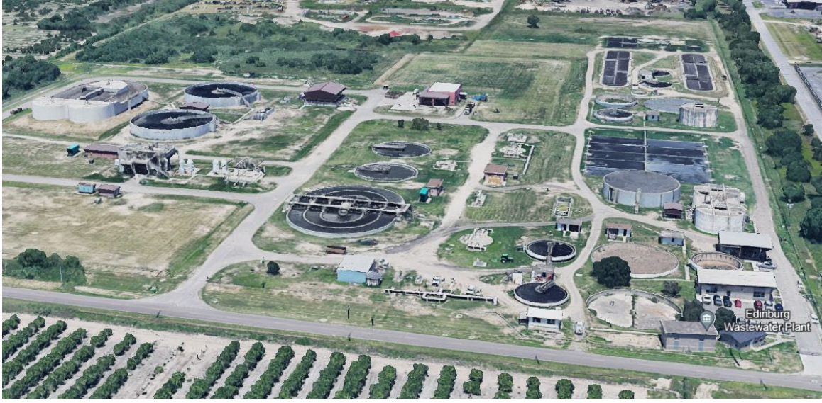
Edinburg Wastewater Treatment Plant - 1202 N. M. Road, Edinburg Texas 78538
