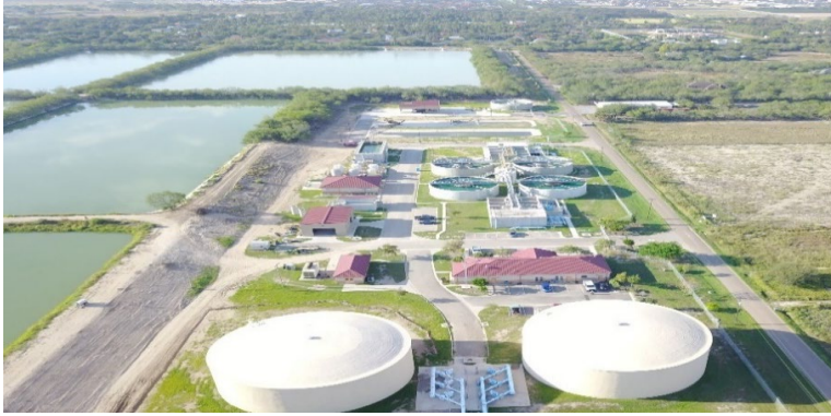
WEST EDINBURG WATER PLANT - 1752 S. MON MACK RD.
