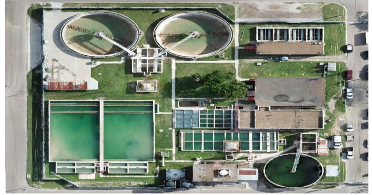
DOWNTOWN WATER PLANT - 500 E. MAHL.
