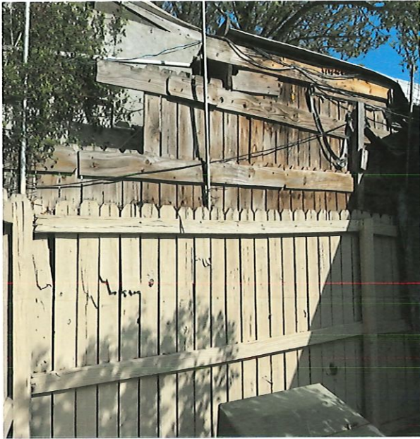
Picture #1 Cracked fence from structure Pushing against fence
