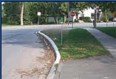
The chicane, raised cross-walk, and curb extension (seen above) are examples of traffic control (or calming) techniques that are achieved through design interventions.
