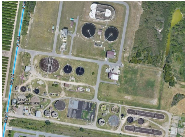
Edinburg Wastewater Treatment Plant - 1202 N. M. Road, Edinburg Texas 78539
