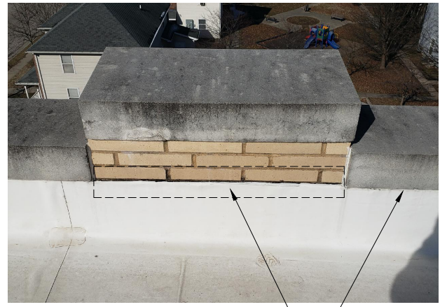
2 A-201 NEW COUNTERFLASHING @ PILASTER (TYPICAL OF 39)
