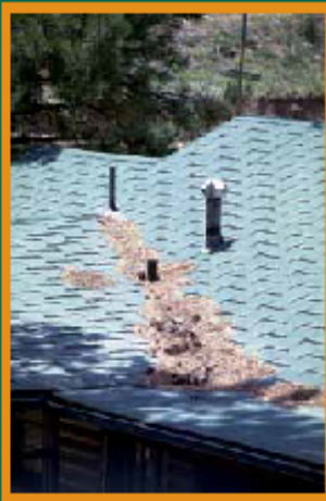
Figure 15: Clearing pine needles and other debris from the roof and gutters is an easy task that should be done at least once a year. Photo: CSFS
