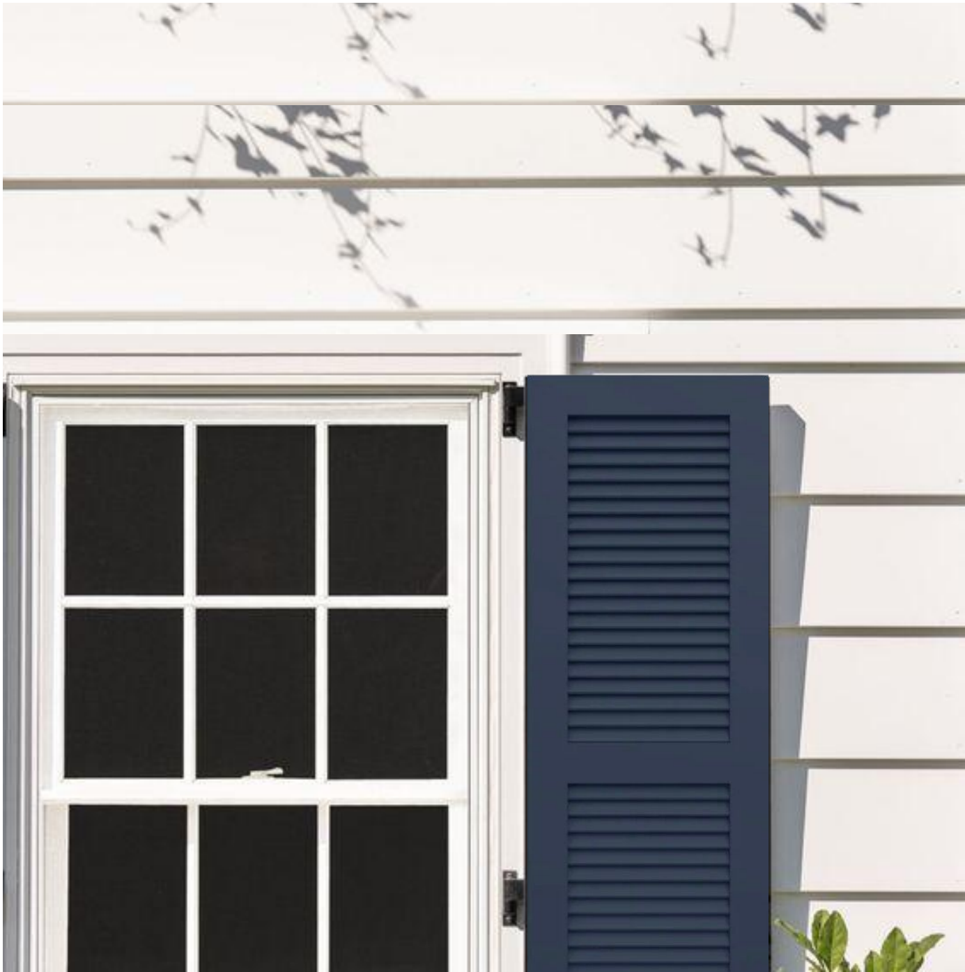
PROPOSED WINDOW TRIM 3 1/2" WIDE WOOD TRIM WITH 1 1/2" SLOPED SILL
