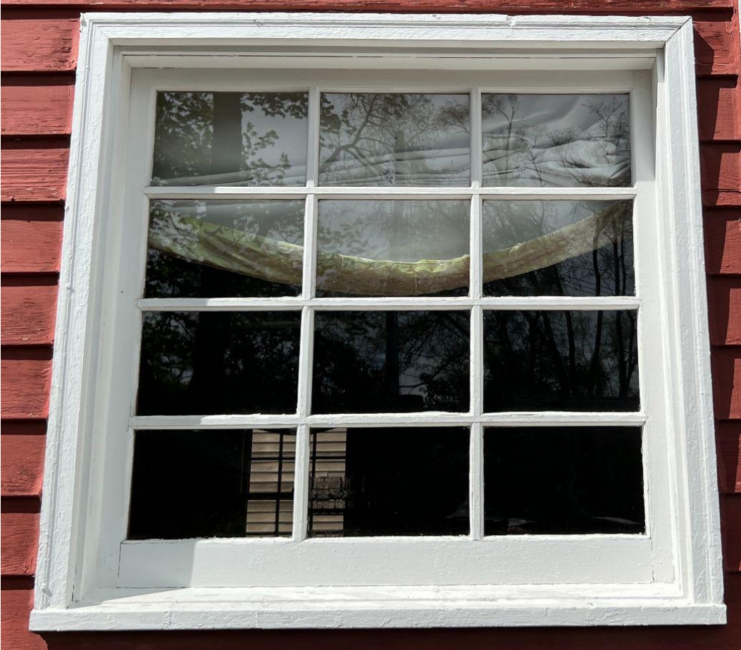
EXISTING WINDOW TRIM 2" WIDE WOOD TRIM WITH 1 1/2" SLOPED SILL
