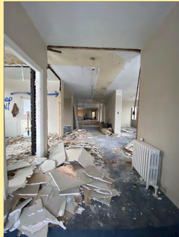
Interior looking east from entry – this will open to a new multipurpose rehearsal, meeting, and recital space with dedicated music teaching studios further east. Ceiling of multipurpose room will be painted open structure. Walls of all spaces are paint finish with LVP in common spaces. Carpet will be used in teaching studios.
