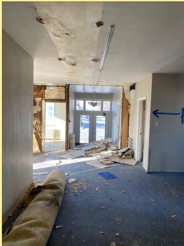
Interior looking west – the north and south corners will be new administrative office facilities. On the south will also be a free snack area. Finishes will be acoustic drop ceiling, paint wall finish, and carpet in offices and LVP in corridor and common spaces.
