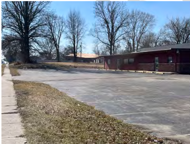
Deteriorated parking lot at 1580 E. Knox Street. (Areas of pavement, which were once asphalt, have receded to lawn.)
