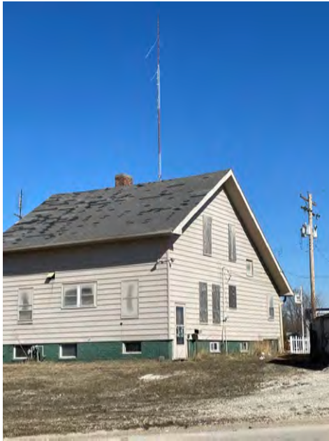
Deteriorated, vacant residential structure (roofing and windows in state disrepair) and site improvements (partially removed building foundation and lack of grading) at 1680 Grand Avenue.
