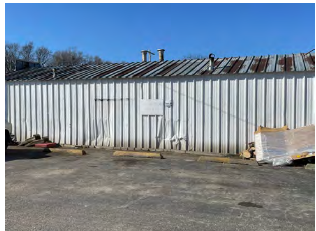
Deteriorated commercial building at 1230 Mulberry Street. (Damaged metal siding and rusted metal roofing.)
