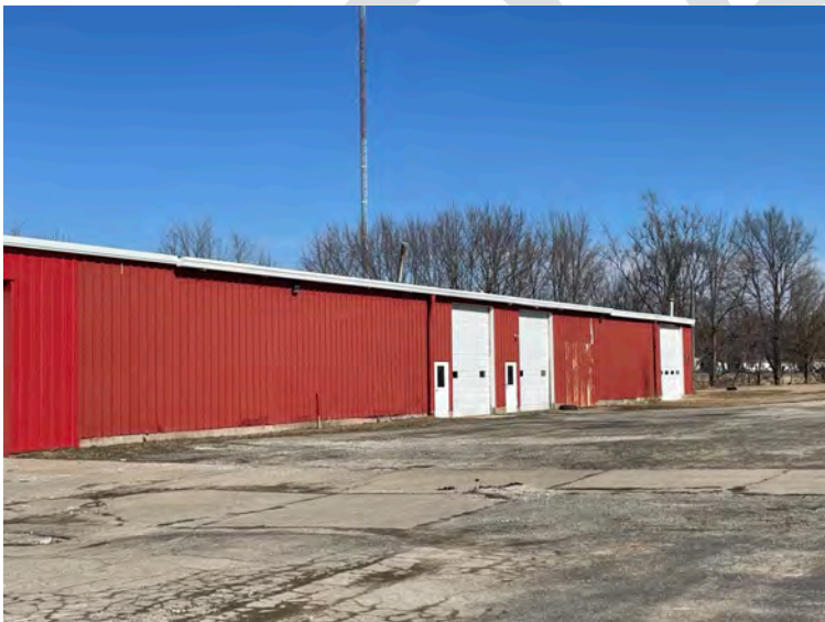
Deteriorated commercial building (damaged metal siding) and site improvements (cracked and crumbling parking lot pavement) at 1611 Grand Avenue.
