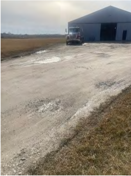
Deteriorated site improvements at 2356 Grand Avenue. (Unimproved dirt and gravel driveway.)
