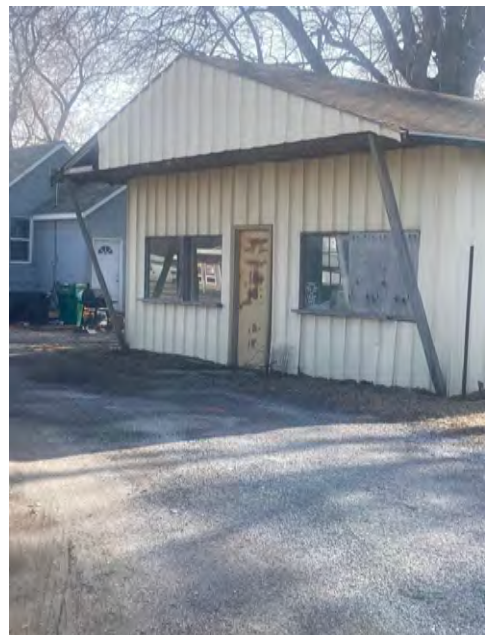
Deteriorated, vacant commercial building at 2400 Grand Avenue. (Missing roof paneling, gutters, broken windows, damaged siding.)
