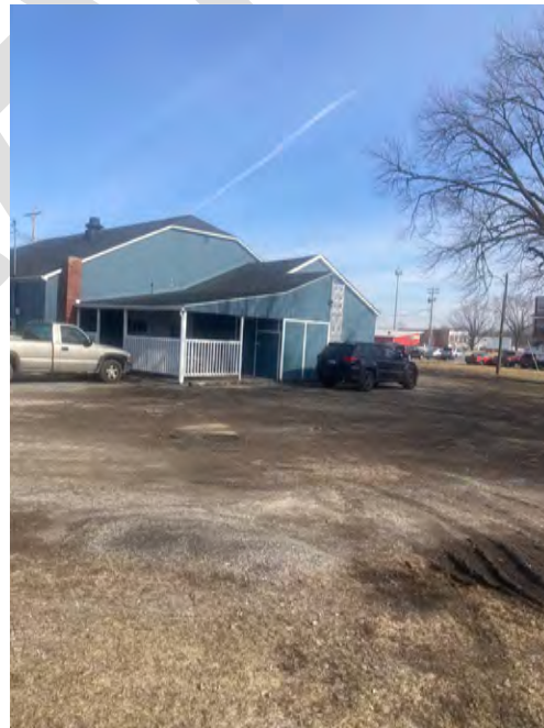
Deteriorated site improvements at 2320 Grand Avenue. (A lack of an improved, dust-free parking surface. Existing dirt and gravel parking surface lacks designated pedestrian and automobile paths. Cars park adjacent to the commercial storefront.)
