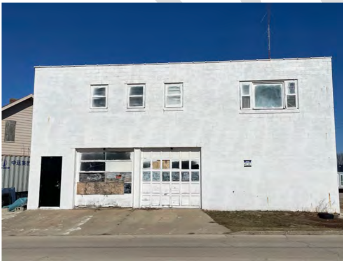
Deteriorated, vacant commercial building (damaged roll up doors, windows, and tuckpointing) and site improvements (cracked and crumbling parking lot pavement) at 1690 Grand Avenue.
