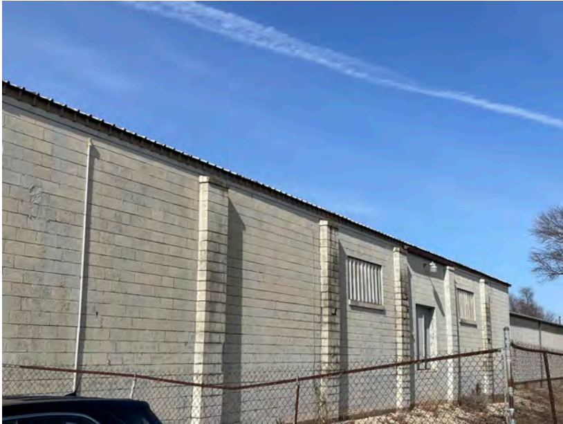
Deteriorated commercial building at 2315 Grand Avenue. (Deteriorating masonry and bowing exterior wall.)
