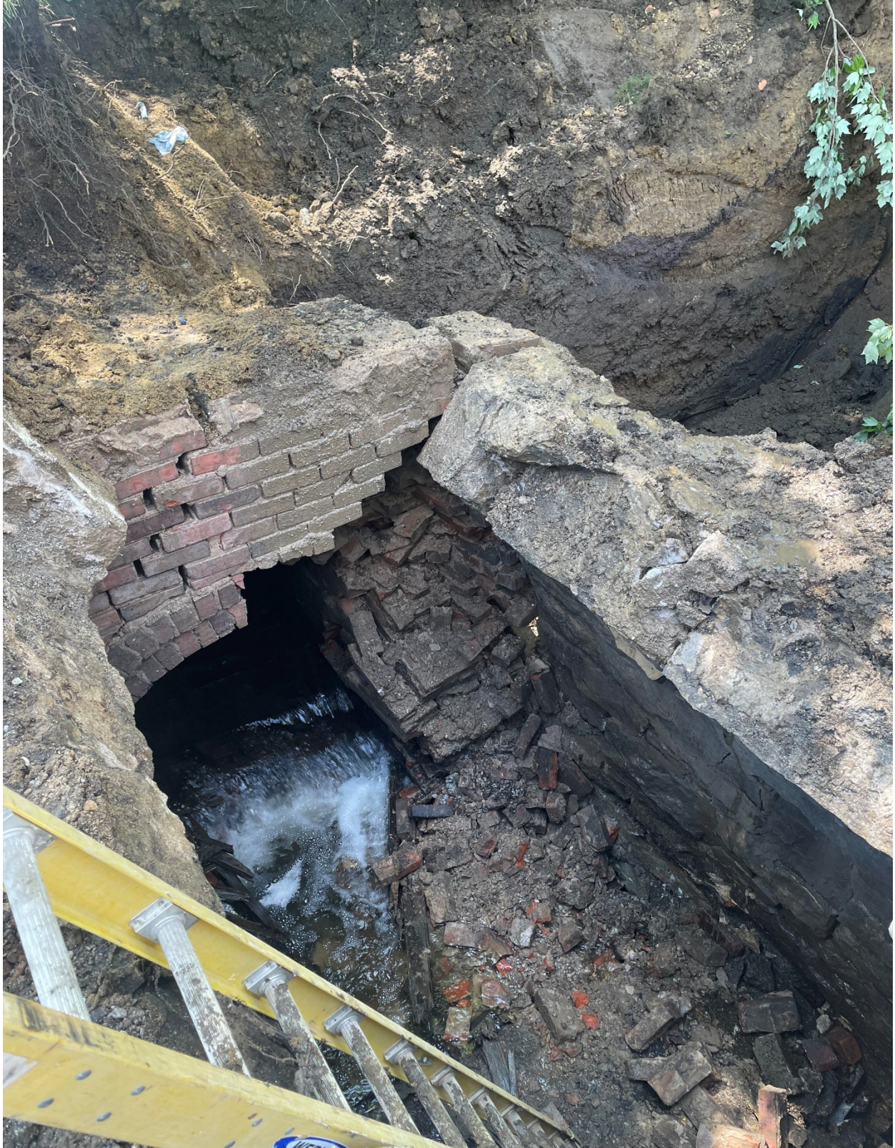
Inside of sewer
