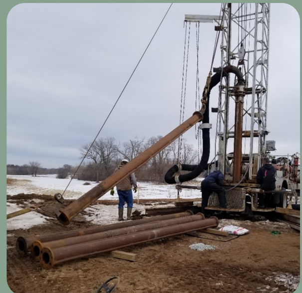
Drilling Gravel Pack Well #6
