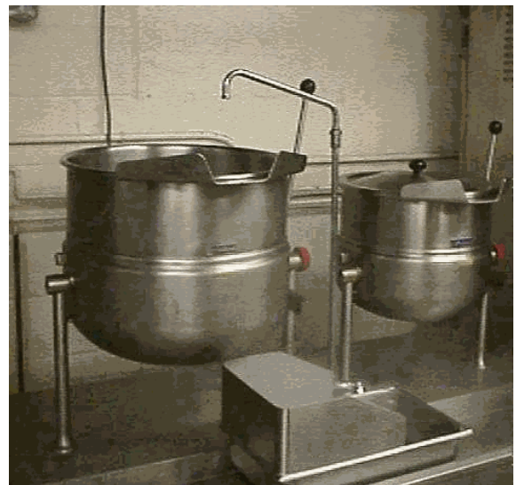
Water Fill to Steam Kettle
