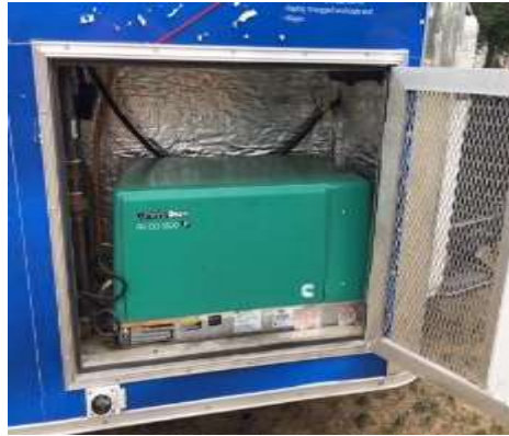
Generator installed in exterior compartment of unit
