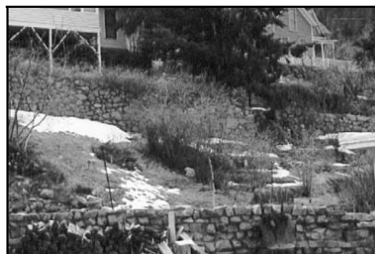
Use earth berms, rock forms or stone retaining walls to minimize visual impacts of cuts.
