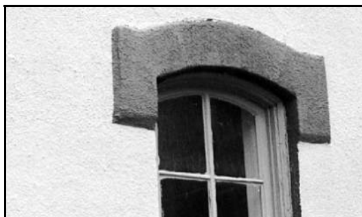
Where a covering of stucco has taken on historic significance, consider repairing damaged areas and periodic cleaning.
