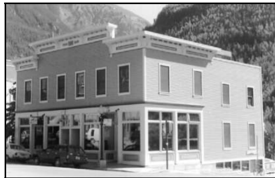
This new storefront is clad in wood siding and uses traditional historic details quite accurately. A stepped cornice expresses the traditional façade widths of the street and upper story windows have traditional trim.
