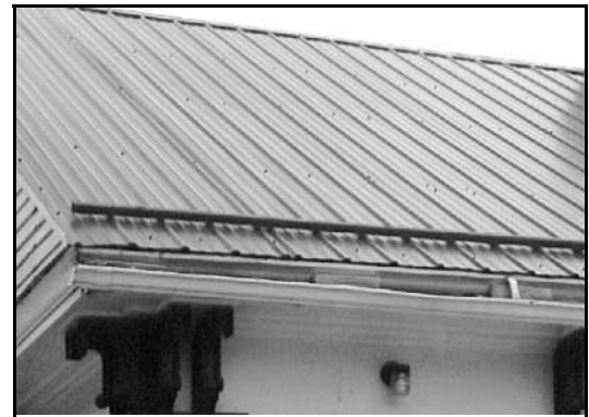
Commercial buildings with metal-clad roofs should have snow guards, brakes or other devices to prevent snow and ice shedding onto public ways.
