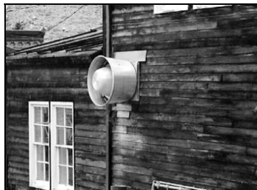
This exhaust fan is not integrated with the building and is inappropriate.
