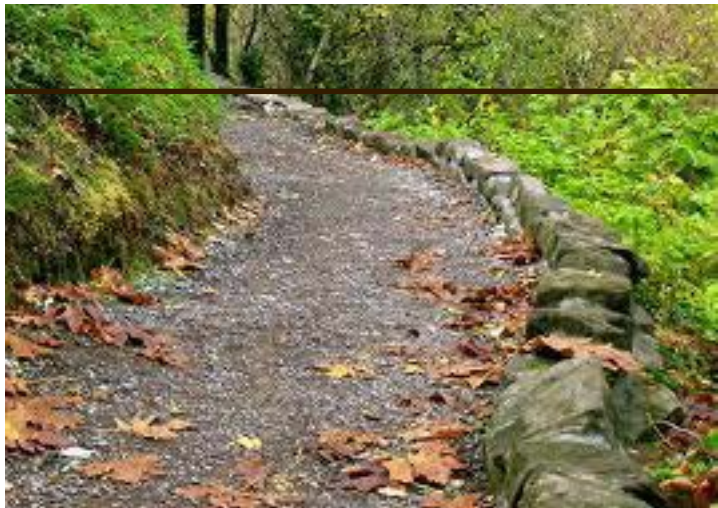
An example of a a crushed gravel trail delineated with a rock edge.
