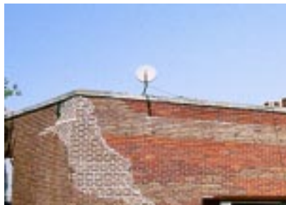
This satellite dish has been properly placed in an unobtrusive place.
