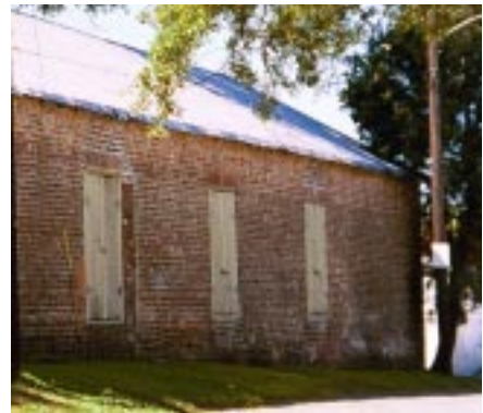
This brick exterior of this warehouse is character-defining and should be retained.
