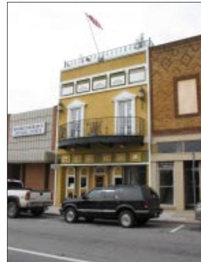
The center building above was inappropriately rehabilitated with added details not original to the building and an inappropriate balcony.
