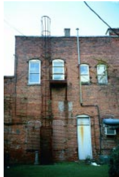
A standard fire escape is located inconspicuously on the rear facade.
