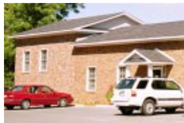
This addition to the rear of the building does not vary by more than ten percent of the height of the original building and it is clear that it is not part of the original building.
