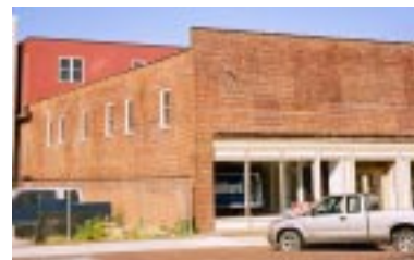
The addition above is correctly placed to the rear of the building and the height is in proportion to the original building.
