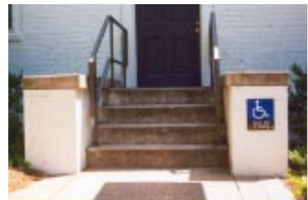
Signage directing disabled persons to a less visible entrance is a suitable design solution.
