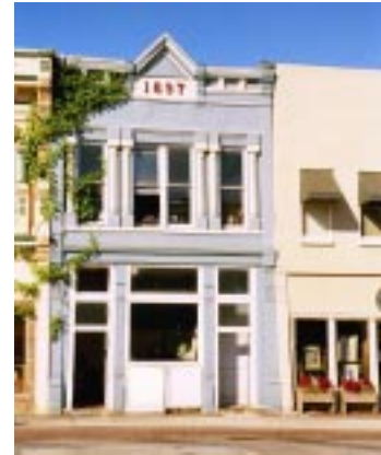
This building's upper story windows are in good repair and are a character-defining feature of this building.
