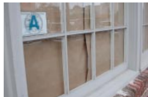
Historic window profiles such as the one seen here cannot be replicated with applied grid systems.
