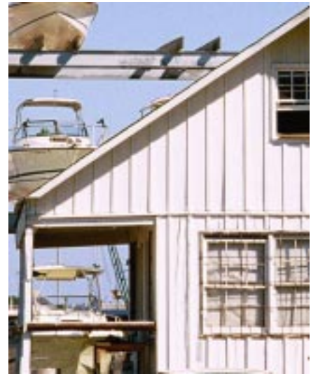
The board and batten exterior of this building is character-defining and should be retained.
