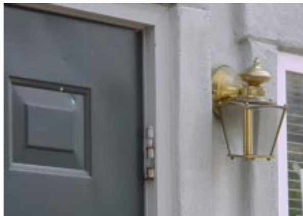
This residential lighting fixture and entrance door are of a style that is not appropriate for the Industrial area.
