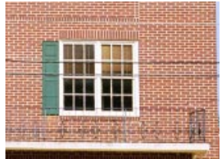
Nonhistoric shutters on this building are inappropriately sized.
