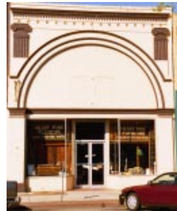
The upper story windows of this building have been covered and now detract from the building's appearance.
