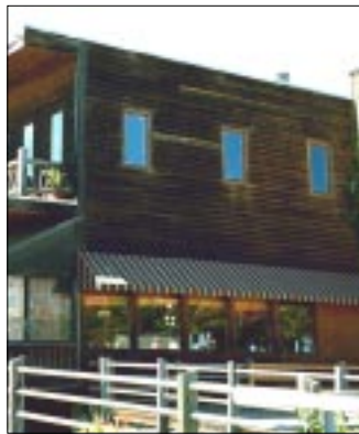
The windows in this building are inappropriate fixed windows that do not maintain the historic character of this building.
