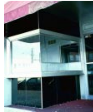
Although not original to the building, this modern storefront has gained significance in its own right and should be preserved.
