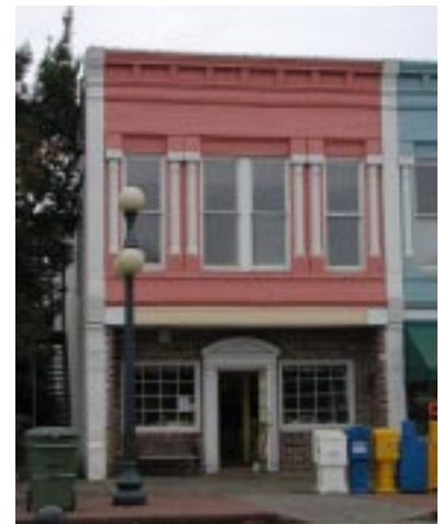
The recessed brick veneer wall and small multi-paned display windows do not reflect the building's date of construction.
