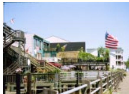
If the above dock area had been made with the same materials and treatments, it would present a more unified environment.
