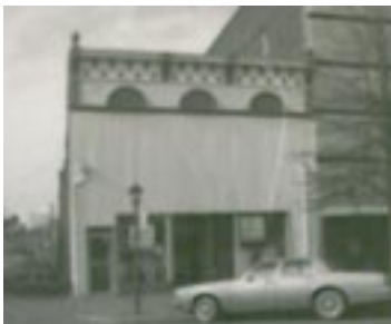
Removal of the aluminum facade (left) facilitated the rehabilitation of this now-contributing storefront in Milledgeville, Georgia.
