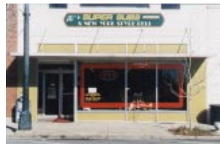
This storefront has been covered with inappropriate materials.
