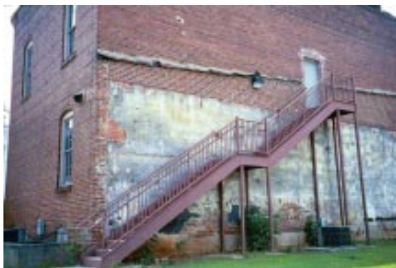
A simple, yet effective solution for a rear fire exit.
