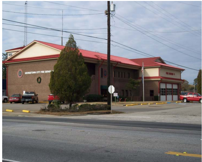
Main Fire Station Located on Fraser and Prince St.
