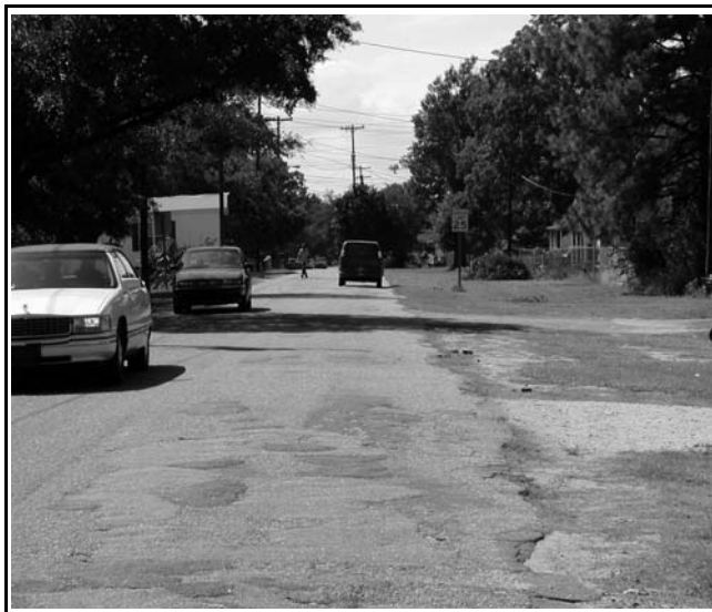
Patching and Poorly Defined Road Edge
