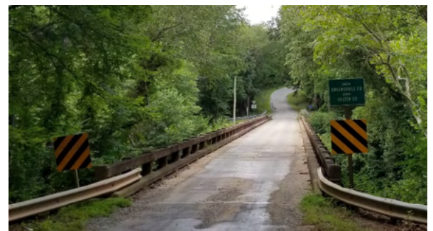
Poor Bridge Ratings (2): -Moonlight Road (616) over Three Creek -Moore's Ferry Road (629) over I-95
