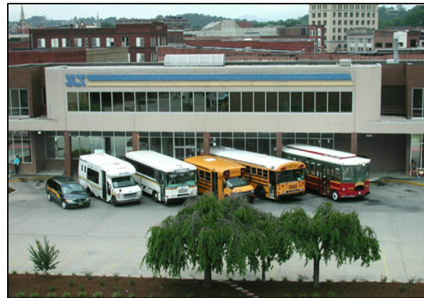
Johnson City Transit Center
