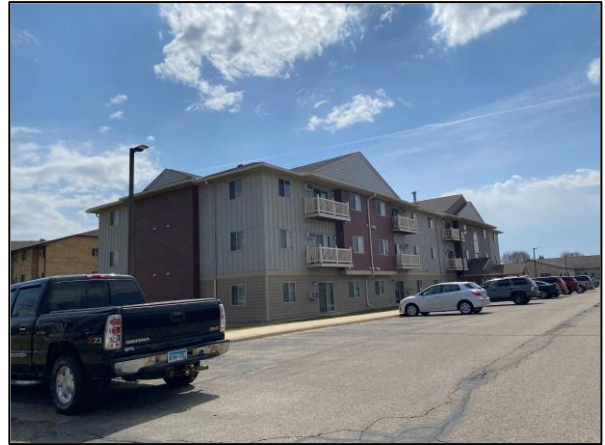
Rozell II Apartments – Dodge Center
