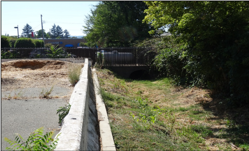
Photo 7: View of 6 th Street storm drain.
