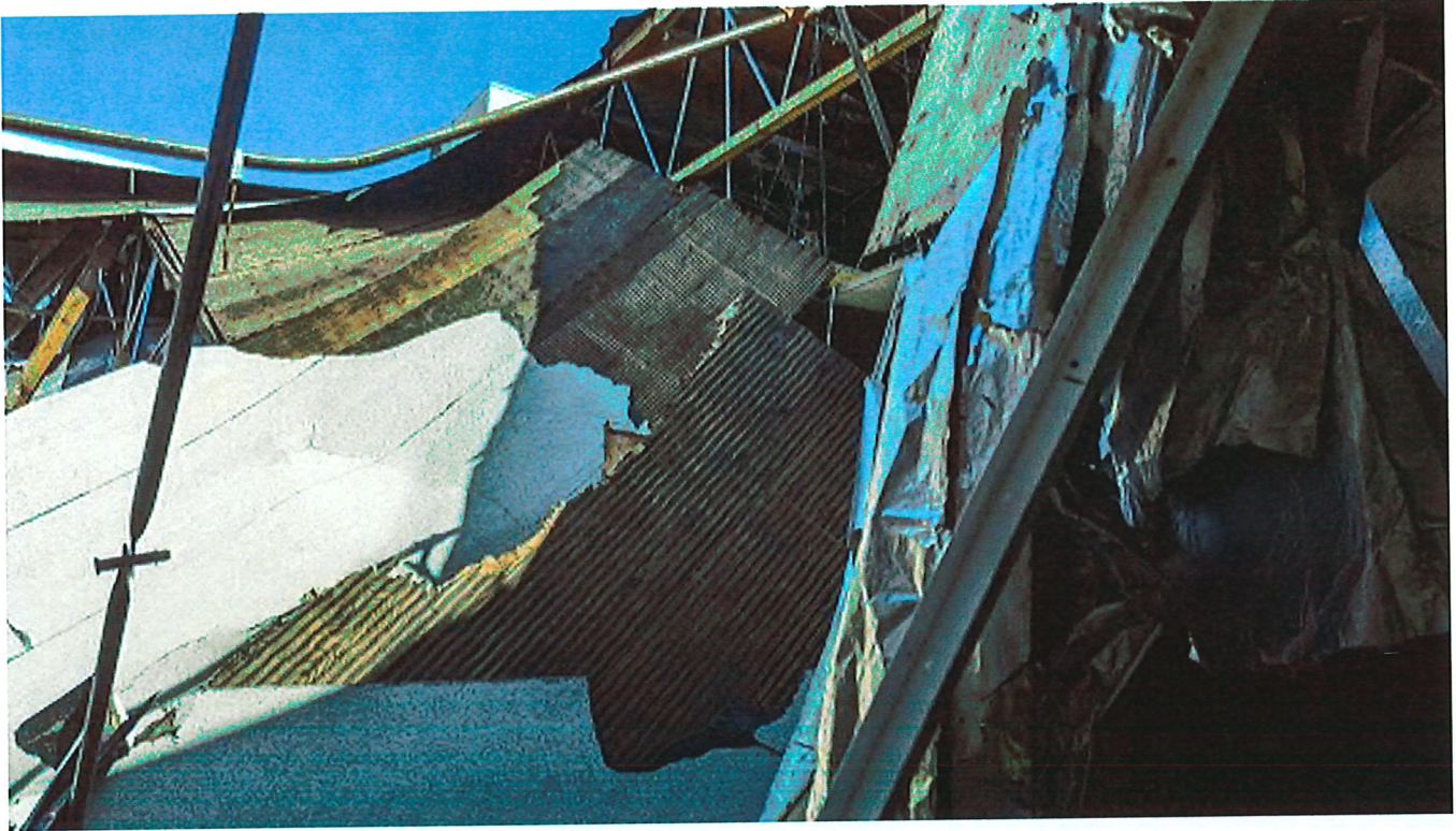
Photo 7 – Plywood decking, Building A
