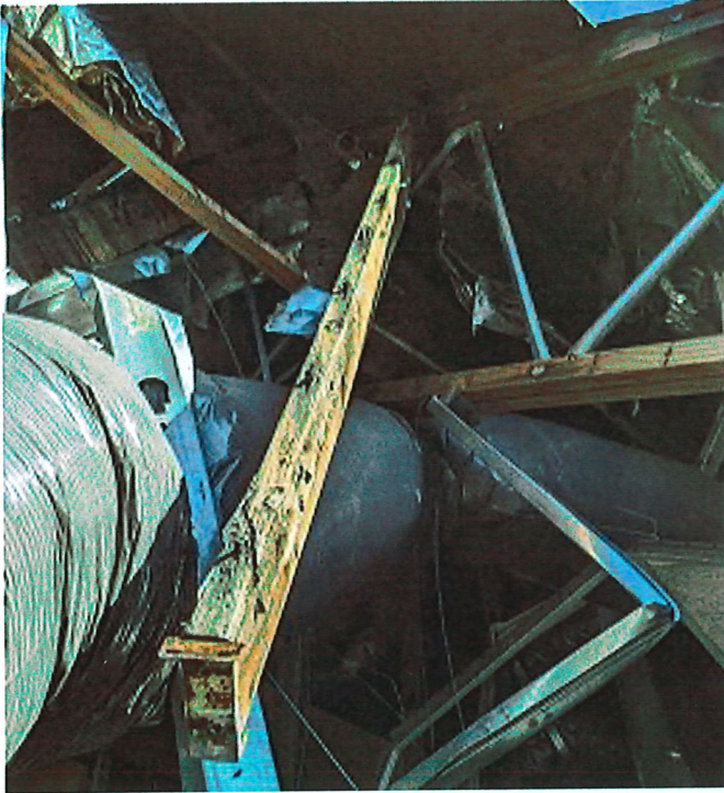
Photo 11 – 2x6 Sub-framing, Building A
