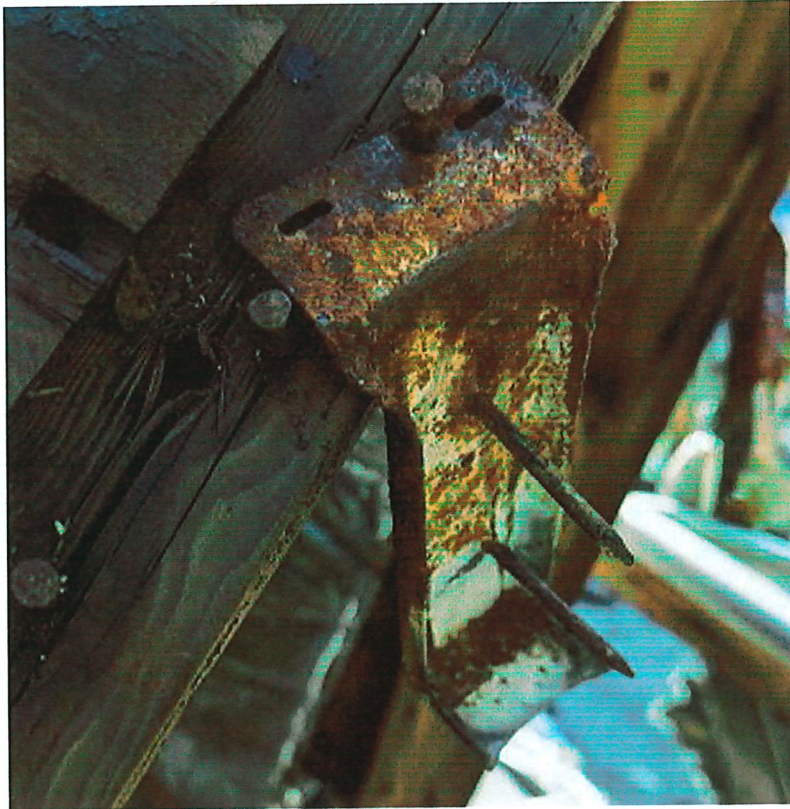
Photo 12 – Sub-framing hanger, Building A
