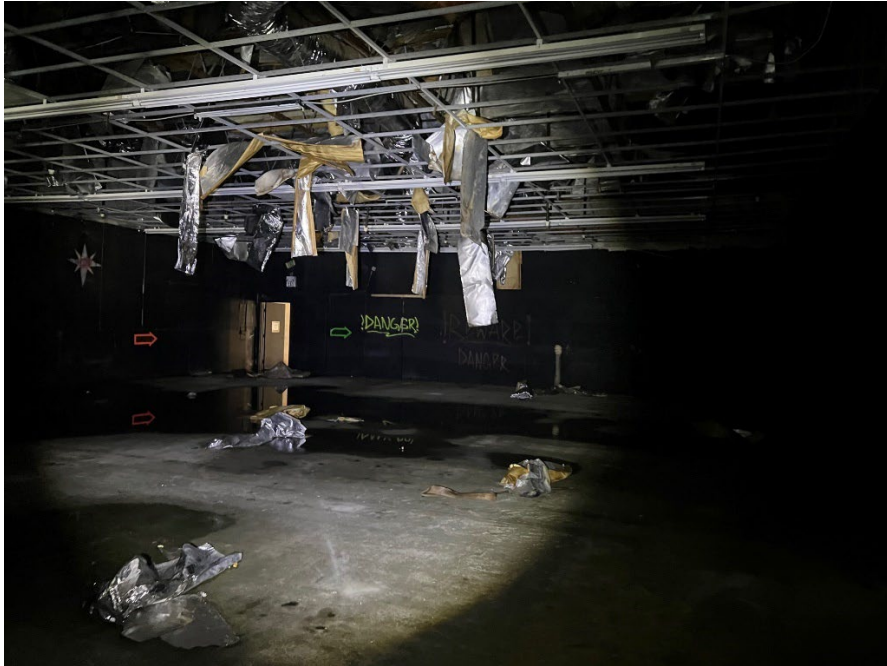
Unit A – Northwest portion of building
