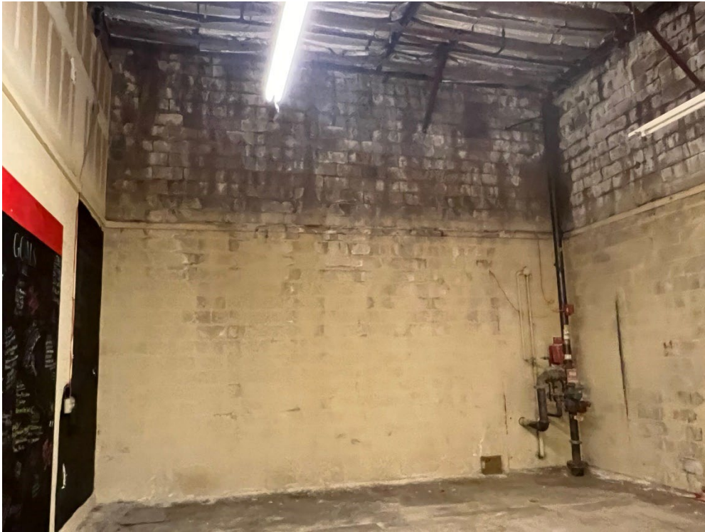
Unit C – North West wall, water intrusion
