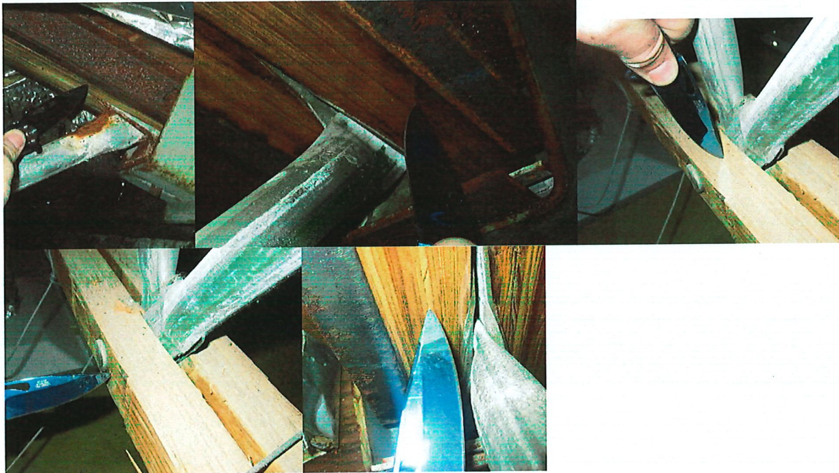
Checked trusses- all spots found with solid hard wood with no water damage. All trusses along this line have 1"x2" "C" channel each side of top chord from the bearing point to the first pin placement 42" from end of truss.
