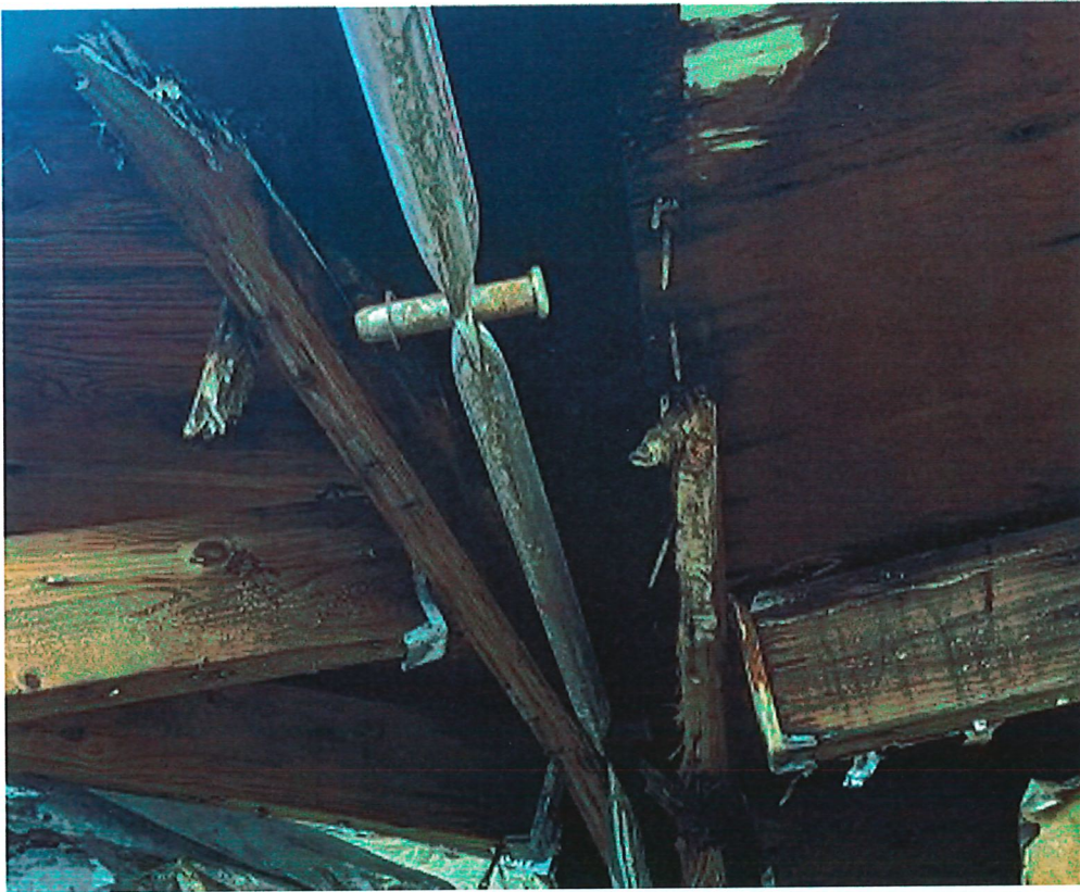
Photo 3 – Steel pin connecting truss diagonals, Building A
