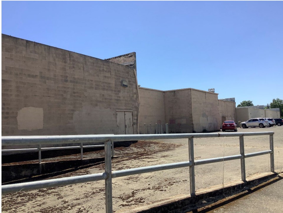
Rear of Units B - G
