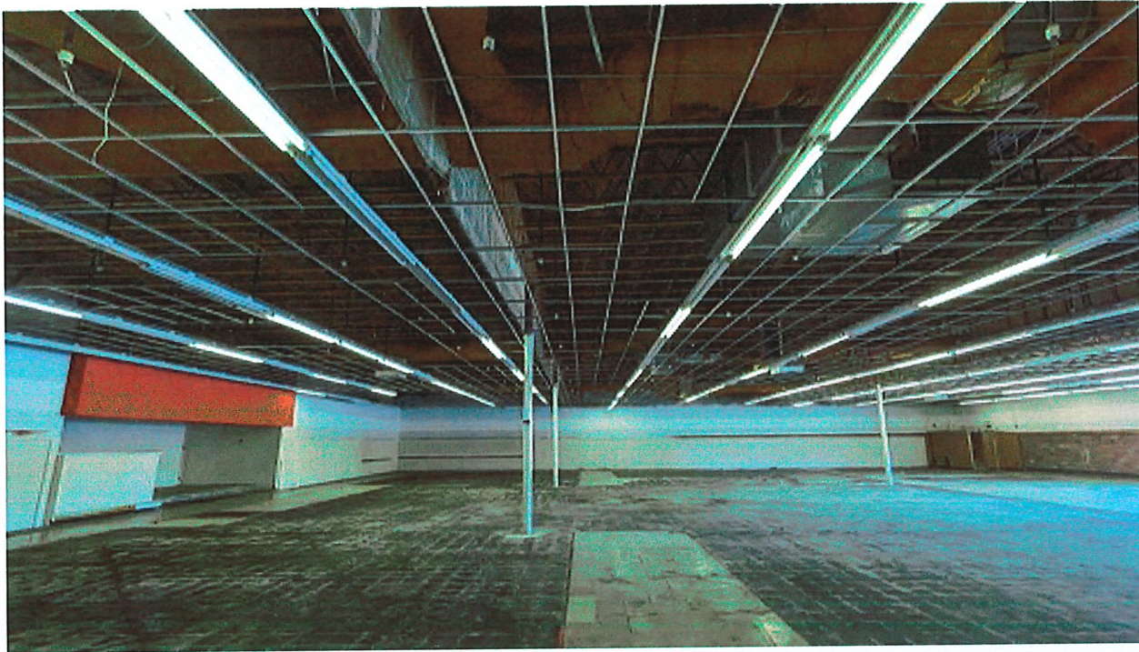
Photo 23 – Main area, Building C
