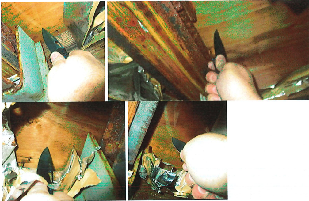
Checked trusses- all spots found with solid hard wood with no water damage. All trusses along this line have 1"x2" "C" channel each side of top chord from the bearing point to the first pin placement 42" from end of truss.
