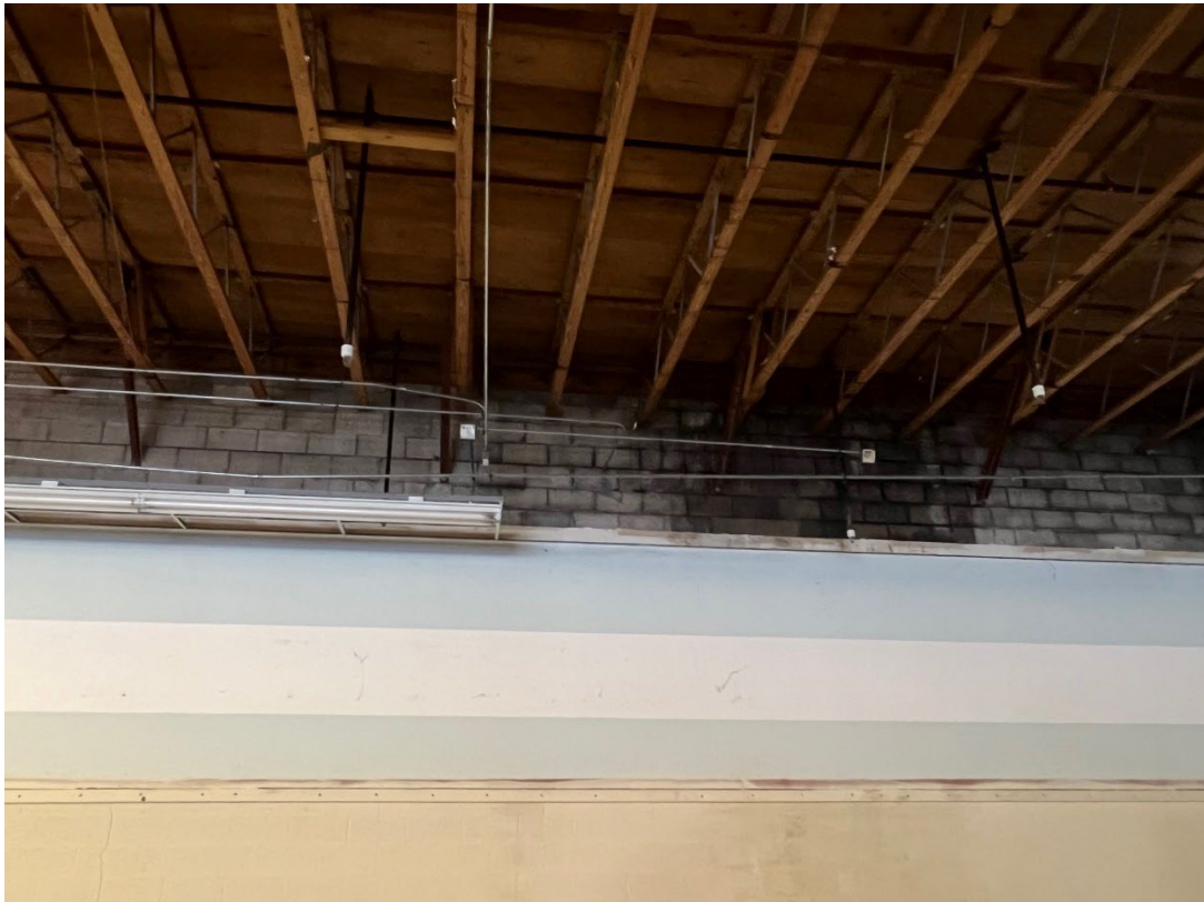
Unit C – North West wall, water intrusion
