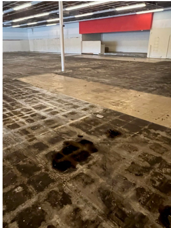
Unit C – Water intrusion in center of unit
