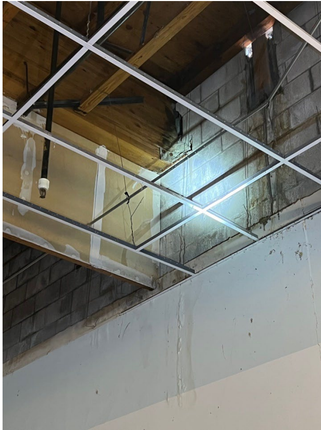
Unit C- Shared wall with Unit B, exposed glulam beams
