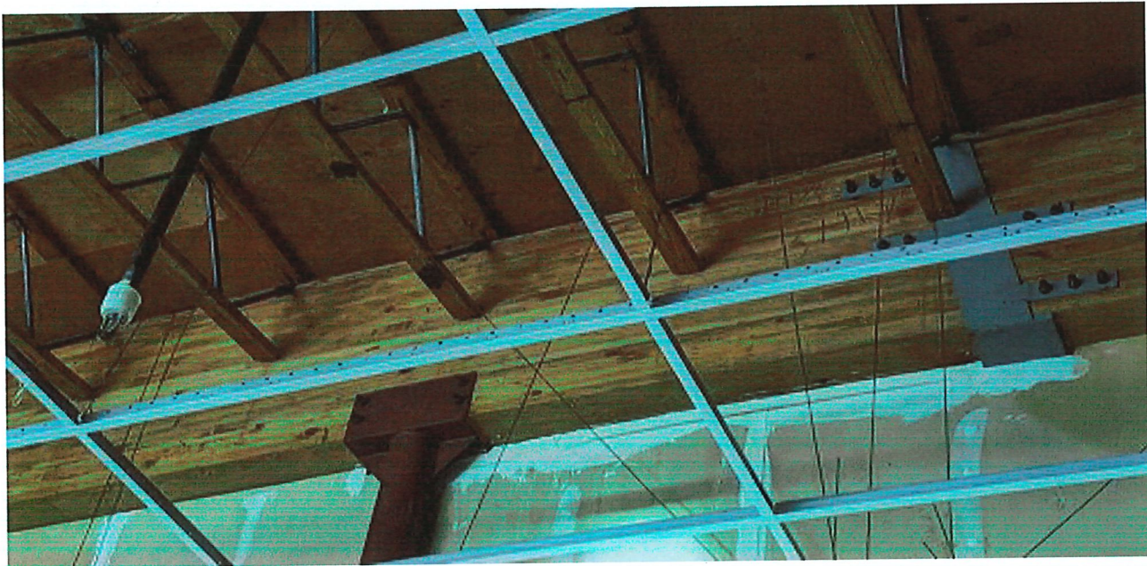
Photo 22 – Typical framing, Building C
