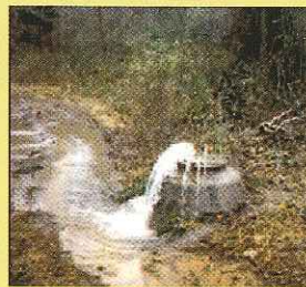
Example of a Sewer System Overflow (SSO)
