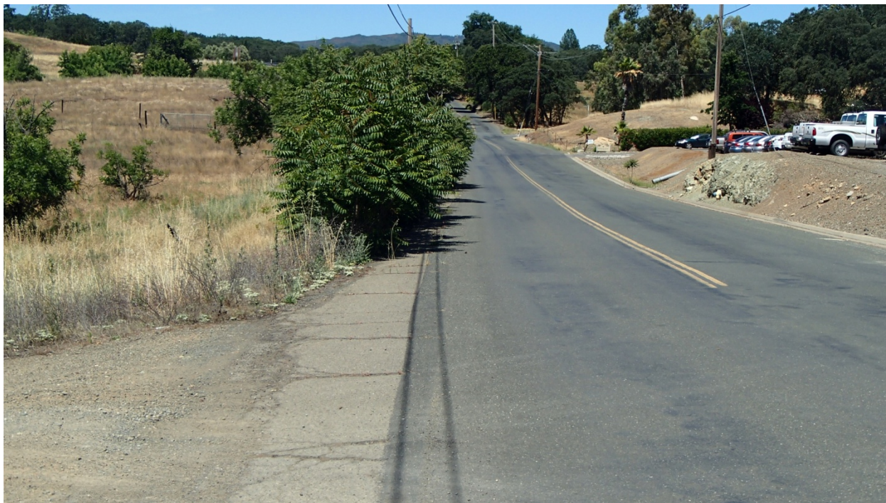
Figure 5: View of Martin Street to the west from the Smith Street intersection depicts sight distance obstructions due to overgrown brush.
