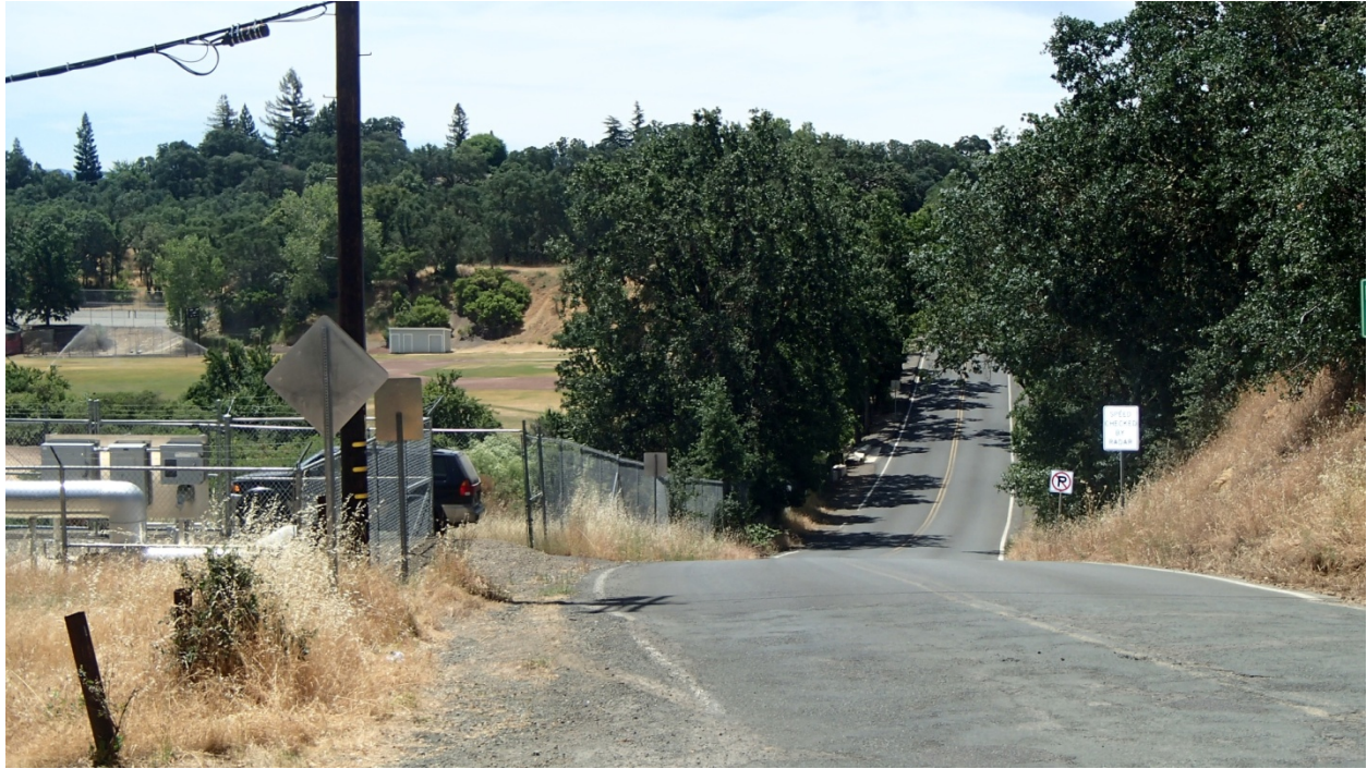
Figure 3: View south along Hartley Street from the north City Limit. Horizontal and vertical curvature depicted here is typical of the entire street segment.
