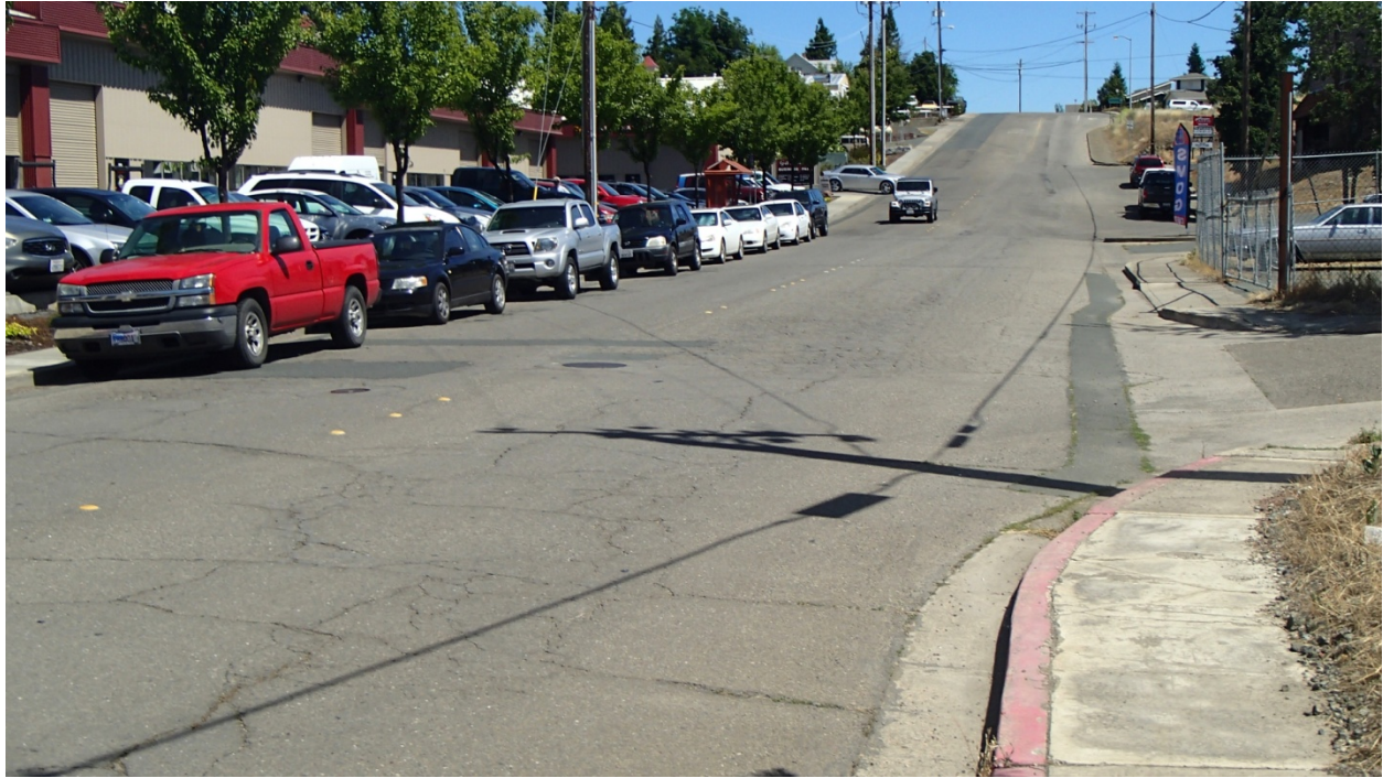
Figure 1: View to north along Bevins Street. On-street parking adjacent to Gateway Business Park constrains southbound travel lane to less than 10 feet in locations.
