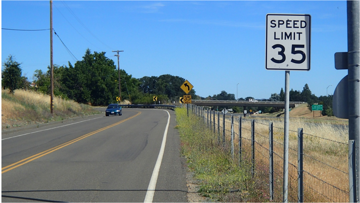
Figure 7: A 35 MPH sign currently controls traffic ahead of a horizontal curve with an advisory 35 MPH speed on Parallel Drive. If this segment of the street were to be zoned in accordance with CVC standards, the new posted speed would be 45 MPH.
