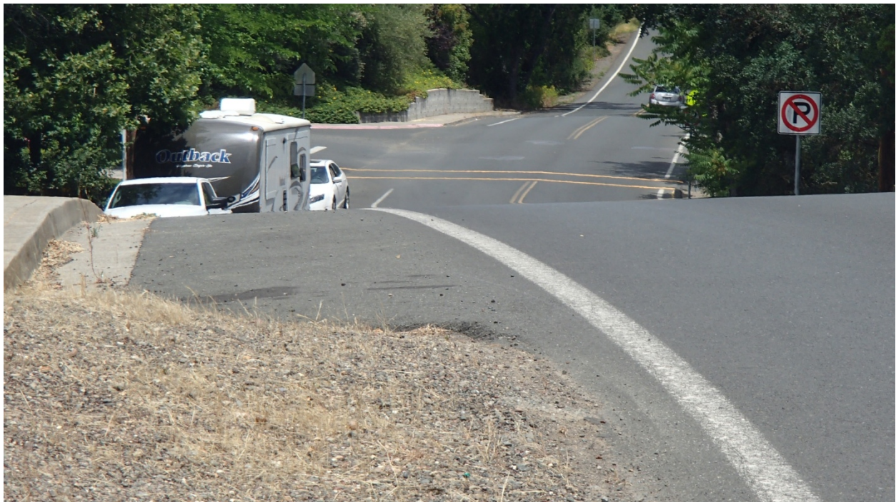
Figure 4: View to the north along Hartley Street. Horizontal and vertical curvature obstructs the view of vehicles and potential pedestrians.
