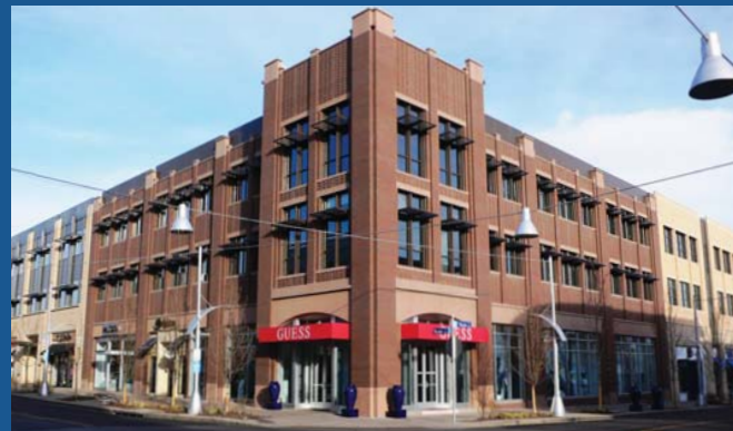
Parapet walls allow mechanical equipment mounted on flat roofs to be hidden from the street level.
