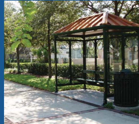
Transit stops should be placed in key locations within an Activity Center in a consistent and identifiable style.
