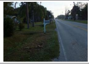
Photo 5: North side of Rosery Rd, looking east. There are no existing sidewalks on the north side of the road. Existing drainage would need to be converted to curb and gutter and mailboxes would need to be relocated along ROW.
