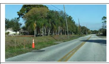
Photo 4: Noted drainage and existing utility constraints that may Possible constraint with extending sidewalk on north impact the construction of a sidewalk along the west side of 58<sup>th</sup> Street.
