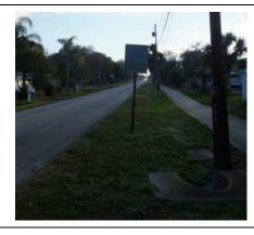
**Photo 3b:**Existing drainage along south side of Rosery Rd. The recommended road reconstruction would convert the existing drainage to curb & gutter.
