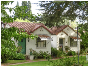
Cottage Court – a group of small detached dwellings facing into a shared court visible from the street
