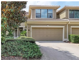
Townhouse/townhome – attached single family homes – limited height compatible with single family detached homes ( see also “rowhome” in Medium-Type definitions below – project team is continuing to refine the differentiation between these two types )
