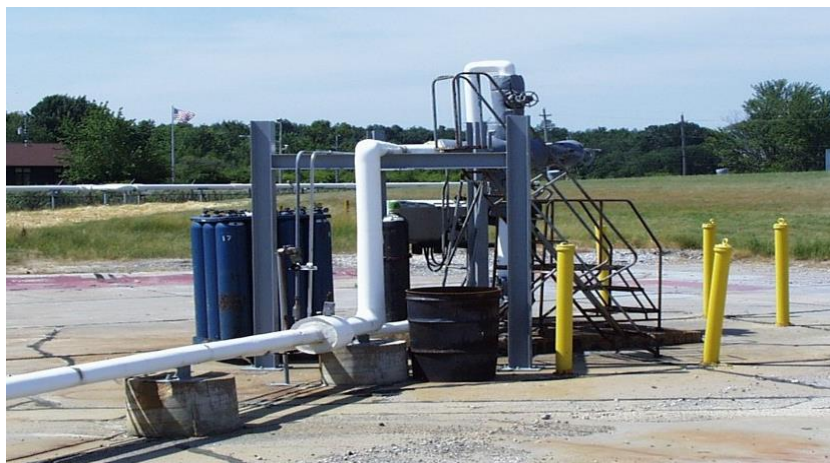
FIGURE 35 – VISUAL OF CLASS 1 INJECTION WELL
