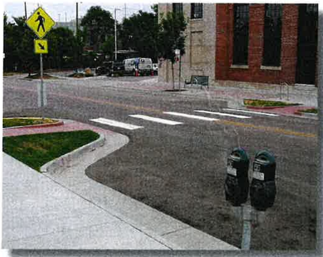
An example of an enhanced street crosswalk featuring bump-outs near on-street parking reduces crossing widths resulting in an increased perception of safety.
