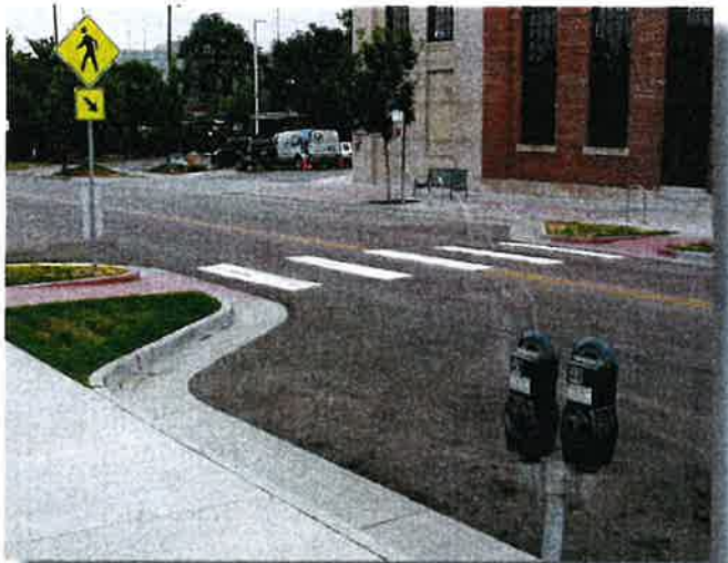
An example of an enhanced street crosswalk featuring bump out, near on street parking reduces crossing widths resulting in an increased perception of safety.
