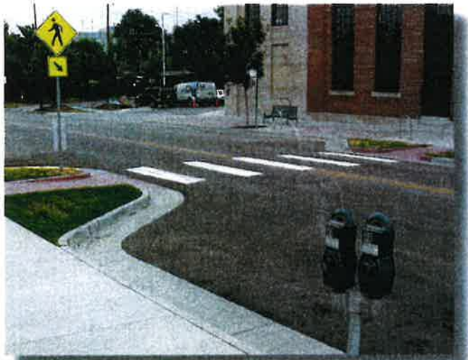
An example of an entrance to street curbside featuring bump-out, near on-street parking reduces crossing widths resulting in an increased perception of safety.
