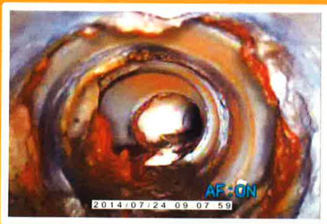
Wall Corrosion: Pitting/Spalling
