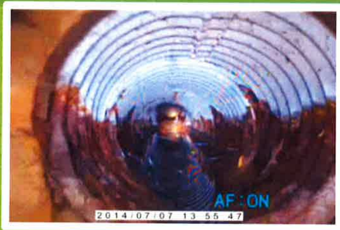
Wall Corrosion: Rough wall
