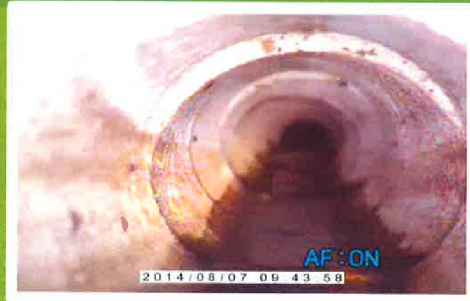
<5% diameter Joint Offset
