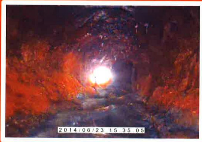
Wall Corrosion: Divots/major spall
