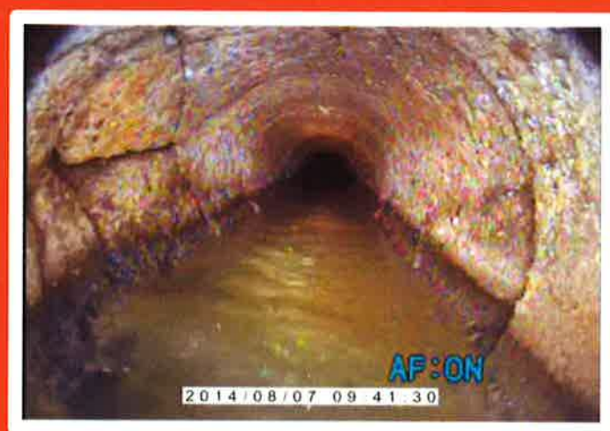
Wall Condition: Extensive cracking
