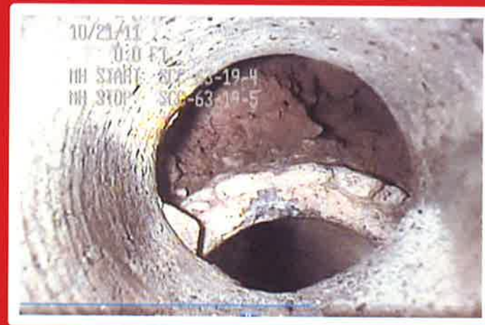
≥ 20% diameter Joint Offset
