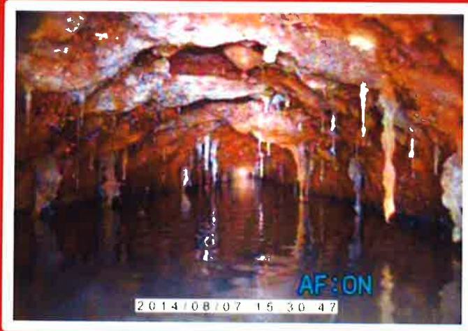
Wall Corrosion: Holes
